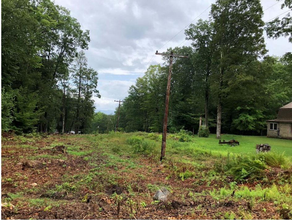
Photograph No. 3: Looking easterly at W110 Structure 2/178 to be replaced.
