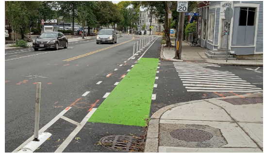
Example of an asymmetrical road diet with two lanes of travel, a separated bike lane, and parking in Somerville, MA
