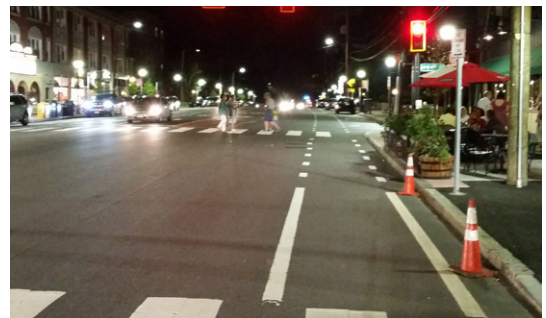
Enhanced lighting example in a commercial district in Arlington, MA
