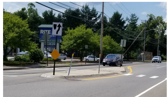
Example of a refuge island in Concord, NH
