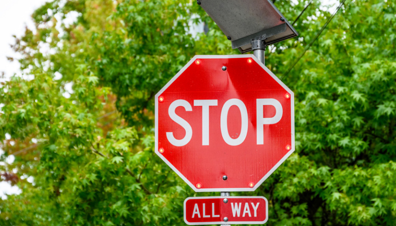
Flashing solar-powered all way stop sign to alert motorist of the upcoming intersection.
