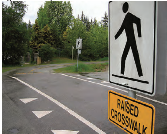
Figure 9 Example of a Raised Crosswalk
