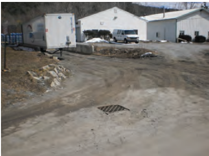
Erosion into Storm Drain on Victoria Street and into Beaver Brook
