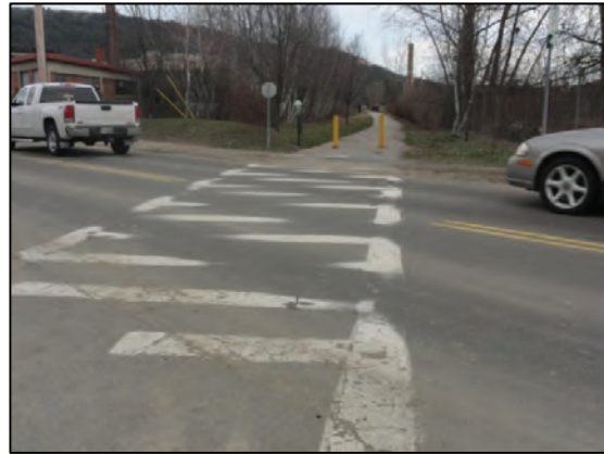
Figure 8 Cheshire Rail Trail and Water Street Intersection
