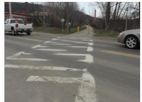
Cheshire Rail Trail Crossing Water Street
