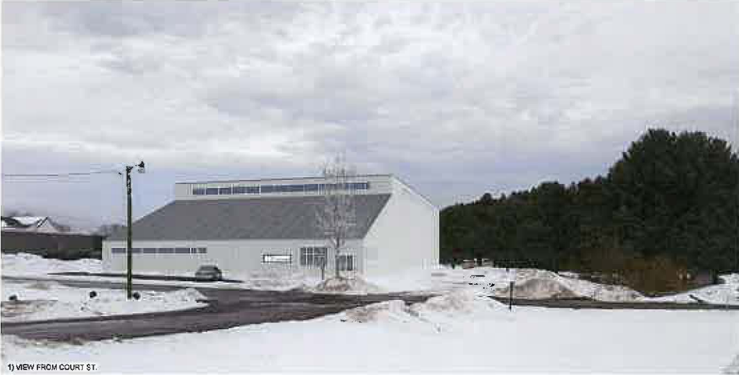
1) VIEW FROM COURT ST.
