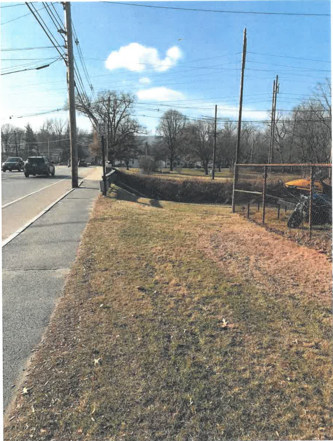
Photo 5 – Northeast quadrant of Winchester Street Bridge (Photo Direction: west)
