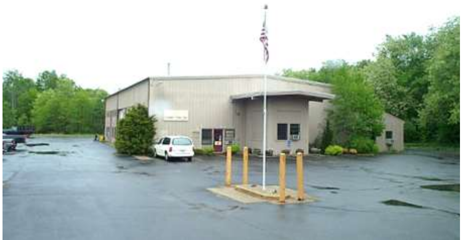
Figure 2: 58 Optical Avenue, Existing Structure
