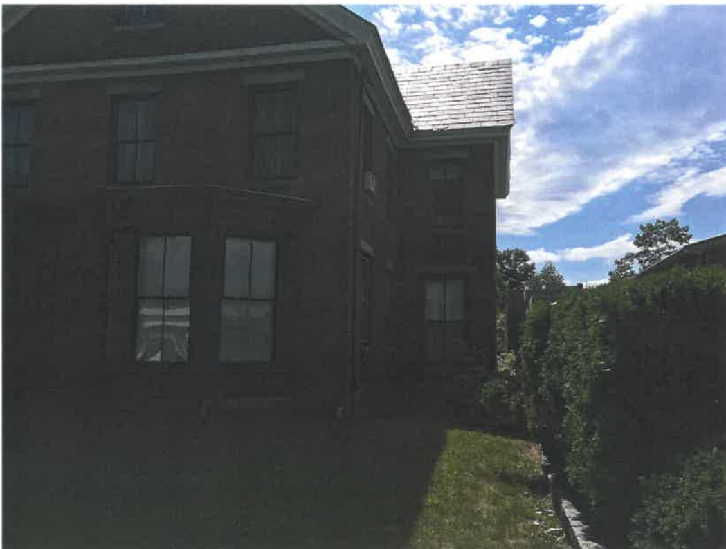
Image of windows to be replaced with woodwork to be repaired and repainted. Also shown is the typical state of the brick that will require repointing.
