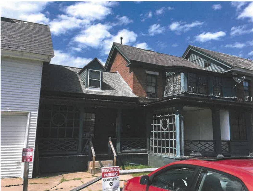
Image of woodwork to be repaired and repainted at side entry and slate roofs to be repaired
