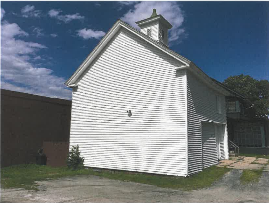
Image of barn to be removed and rebuilt
