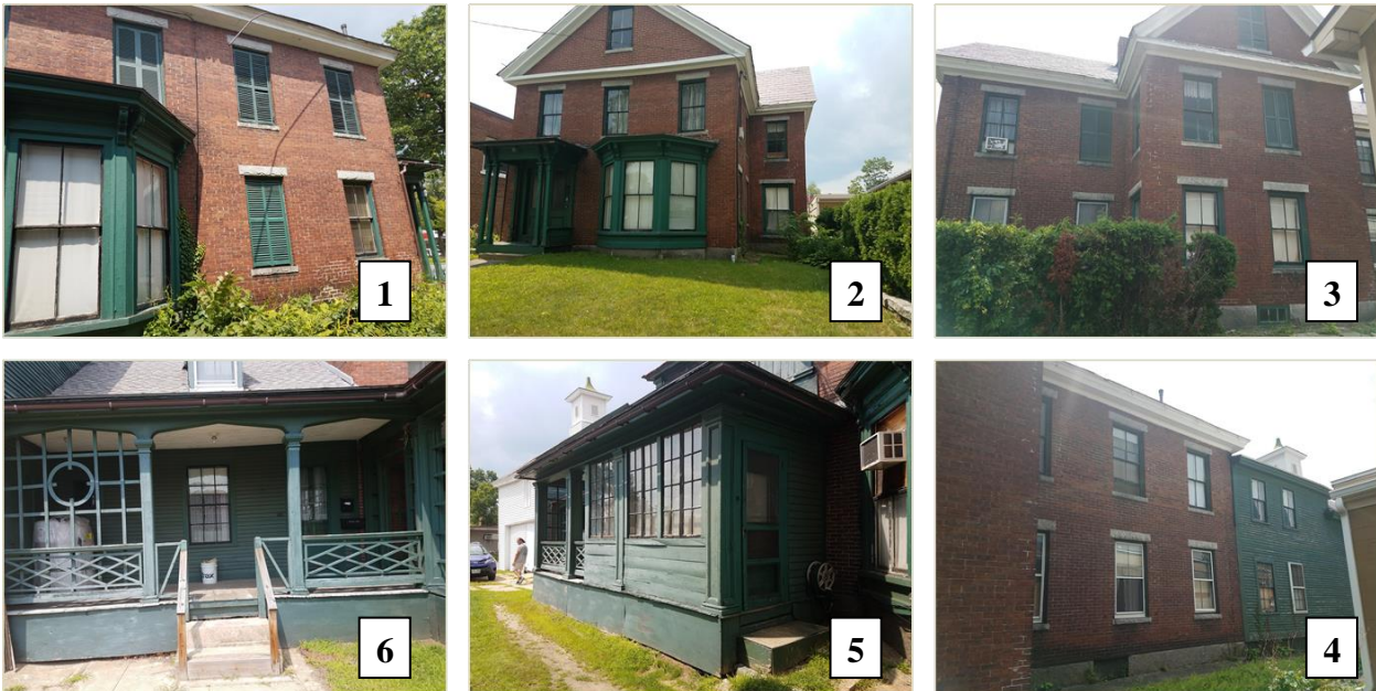
Clockwise from top left: 1 - South façade of building closest to Main Street, 2- East façade of building facing Main Street, 3 - North façade of building closest to Main Street, 4 - North façade of building further from Main Street, 5 - View of porch area on south of building, 6 - View of porch entrance.
