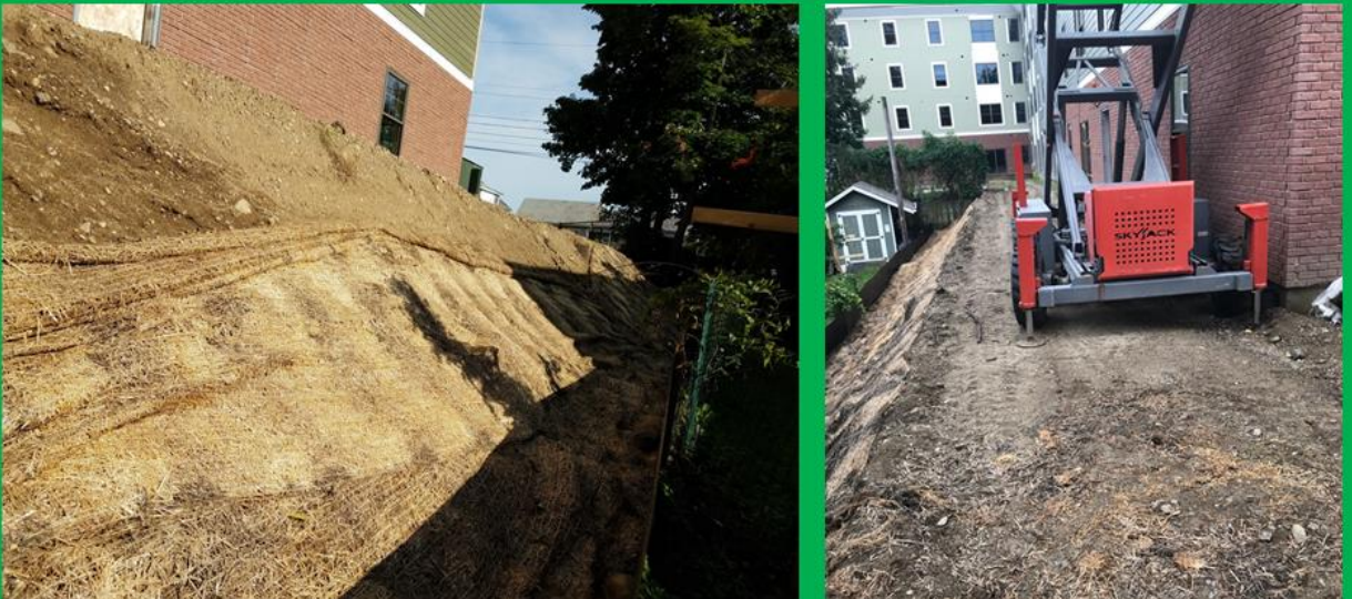
Northeast corner of property adjacent to 47 Spring Street in July 2018, with fill added to create a 2:1 Slope.
