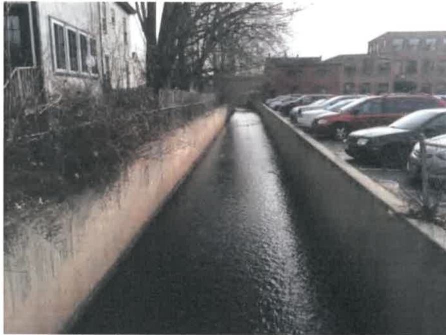
Photo 3 – Facing Beaver Brook downstream from the bridge. Photo taken on 11/30/2017.
