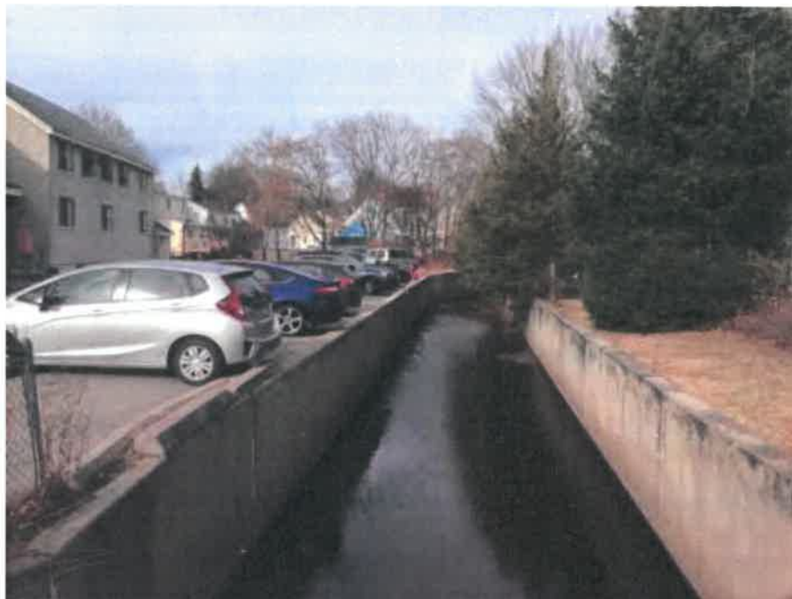
Photo 4 – Facing Beaver Brook upstream of the bridge. Photo taken on 11/30/2017.
