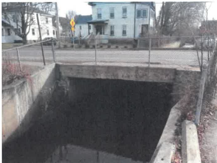
Photo 2 – Facing upstream toward Bridge 192/106 and Impact Locations A, B Photograph taken 11/30/2017.
