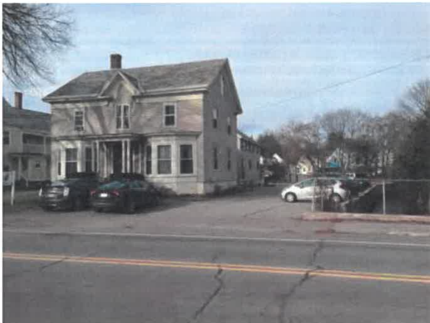
Photo 6 – Adjoining property to the northwest (upstream, western side of the bridge). Photo taken on 11/30/2017.
