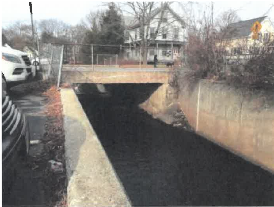
Photo 1 – Facing downstream side of Bridge 140/077. Photograph taken 10/13/2015.
