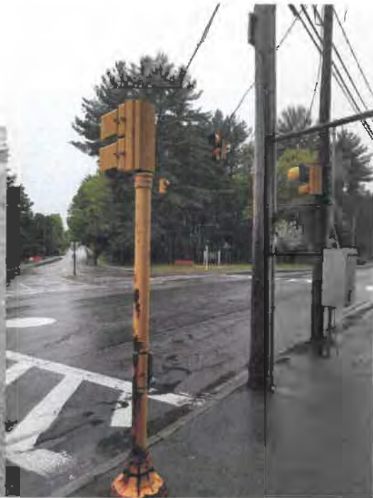
Overall Intersection (view NW)
