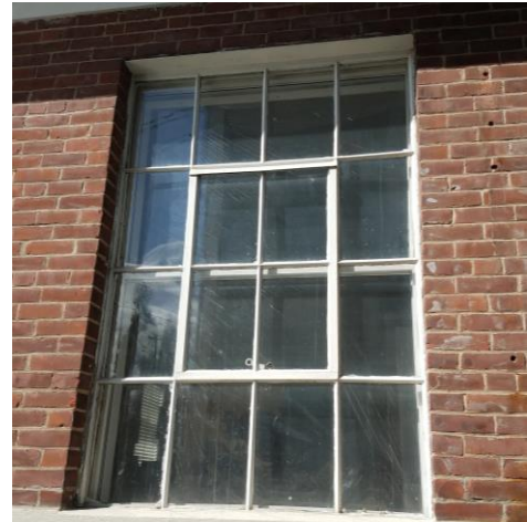
Above: Photo of existing window at 27 Mechanic Street, taken May 6, 2019.
