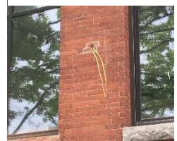
Above: The 6" diameter penetration for ventilation; Below: Penetration for light fixtures.
