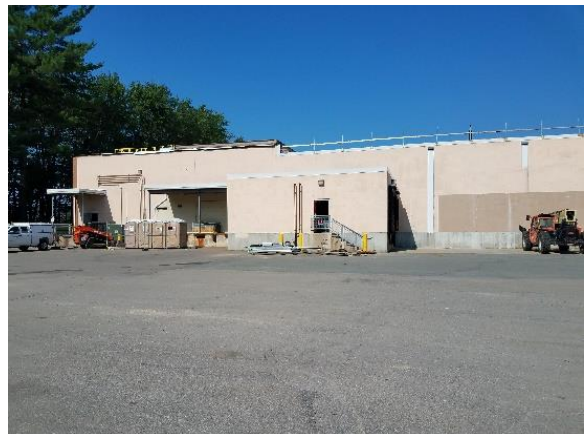
Figure 2. Photo of the rear of the building where a new loading dock and trash compactor is proposed.
