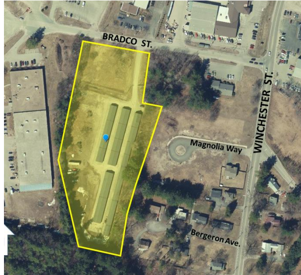
Figure 1. Aerial view of 12 Bradco Street (highlighted in yellow).
