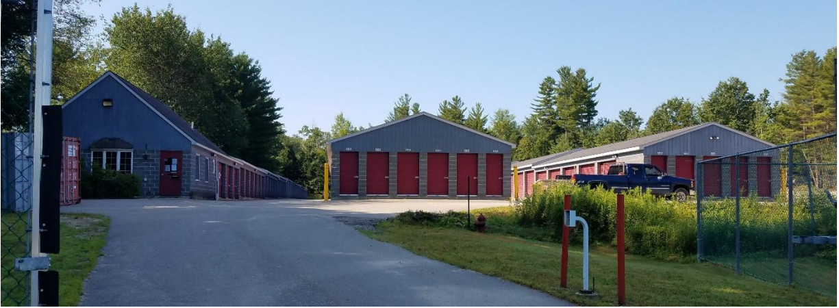
Above: An image of existing CMU buildings on the site. Photo taken August 12, 2019
