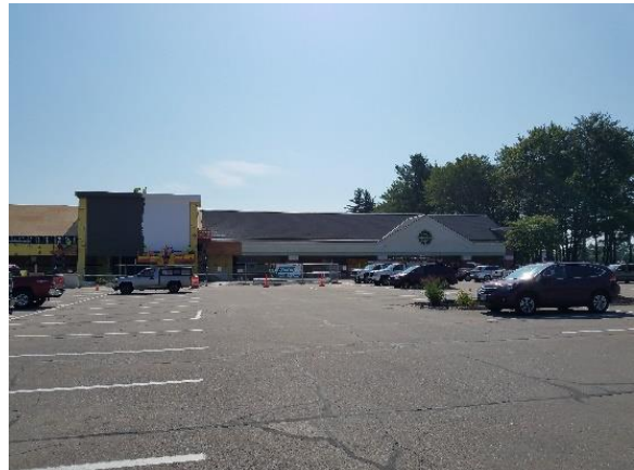
Figure 1. Photo of the existing facade for Tenant Spaces C and D (taken August 6, 2019).
