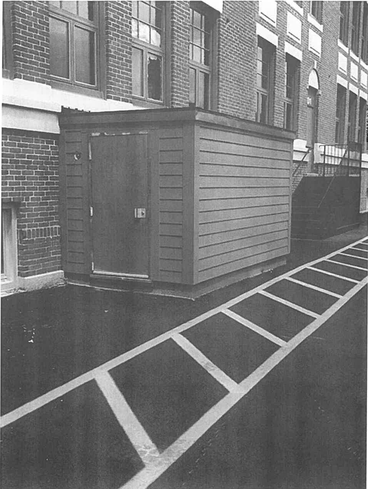
Resided and painted entrance and replaced stair
