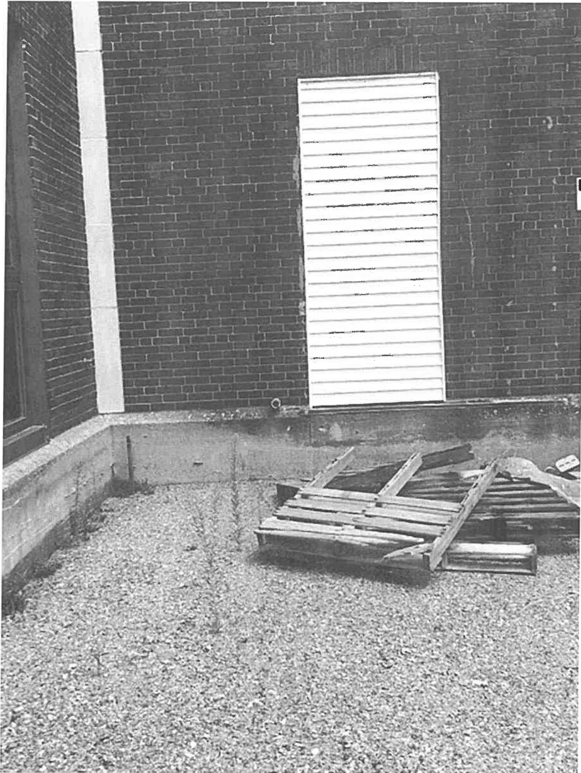
Pipe for Sprinkler drain
