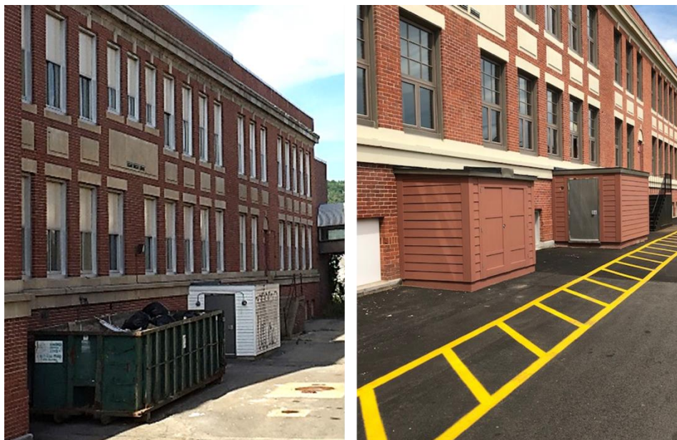
Figure 3. Images of the south side of the former Middle School from 2016 (left) and 2019 (right).
