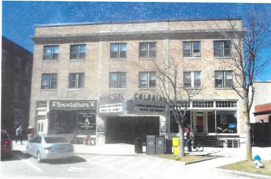
Figure 1 – Colonial Theater Main Street façade today
