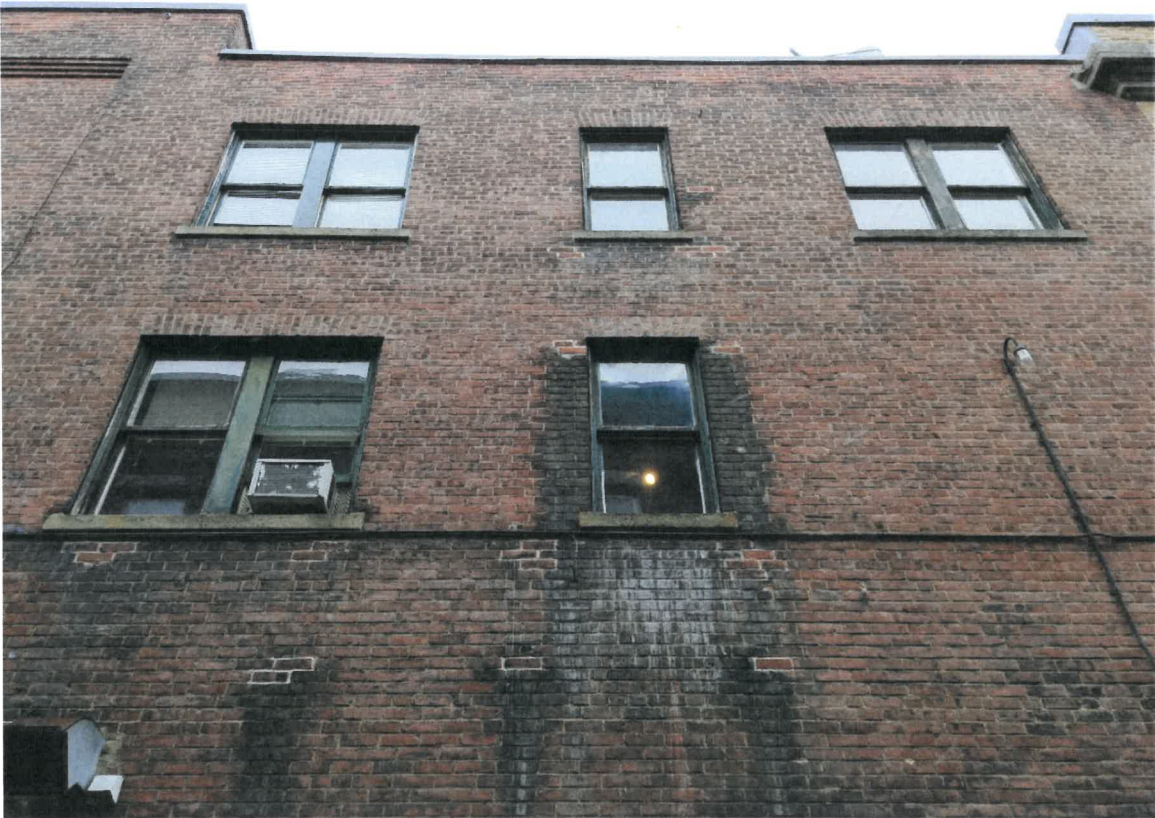
Figure 7 - example of brickwork to be cleaned
