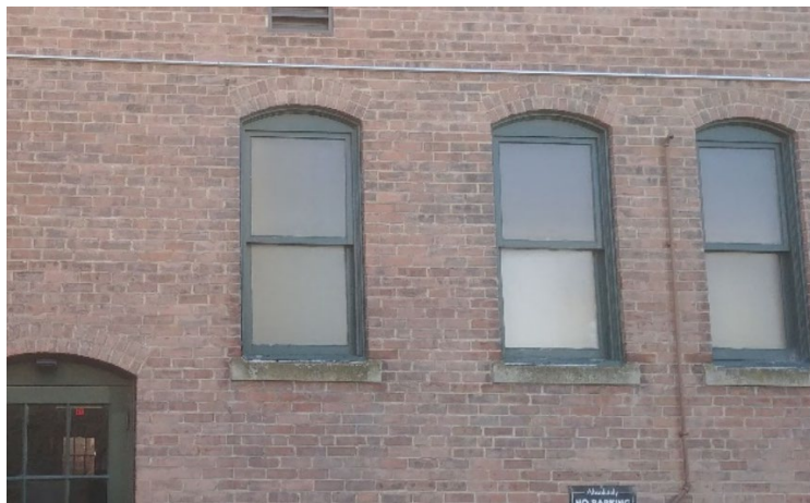
Attachment # 6 - Northside Windows to be Replaced
