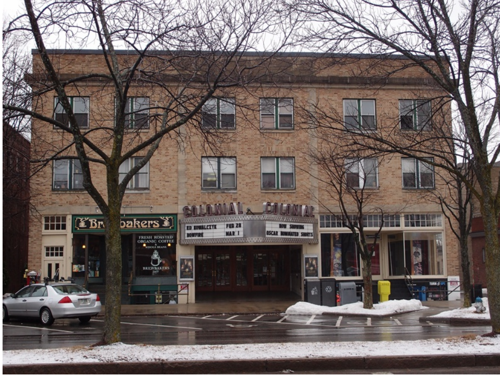
Attachment # 7 – Main Street Windows to be Replaced
