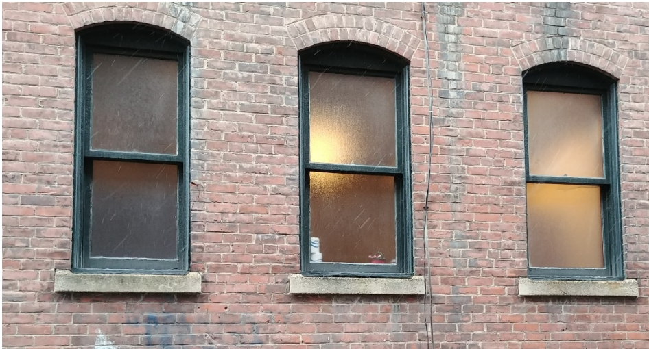
Attachment # 5 - Southside Windows to be Replaced
