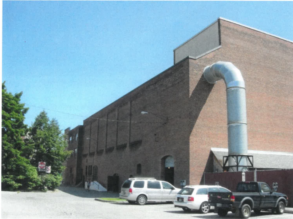
Figure 8 – Existing Stage House view from public parking
