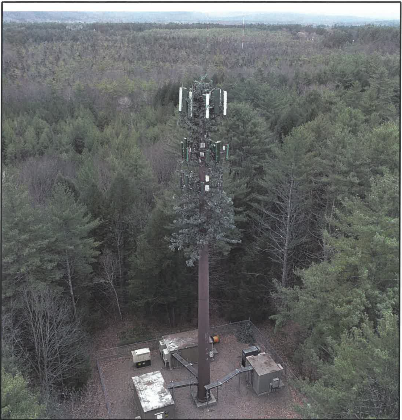
Photo 1—AERIAL VIEW EAST TOWARD PROPOSED COLLOCATION SITE
