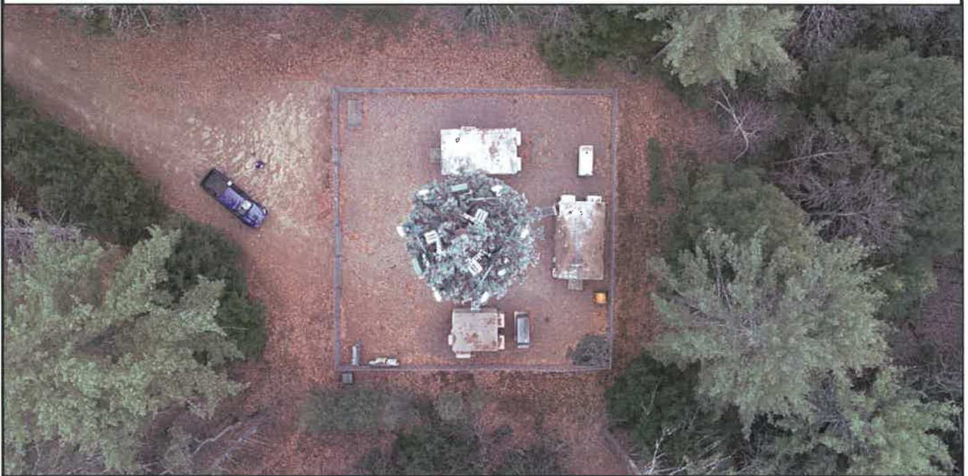
Photo 4 - AERIAL VIEW OF EXISTING TOWER COMPOUND
