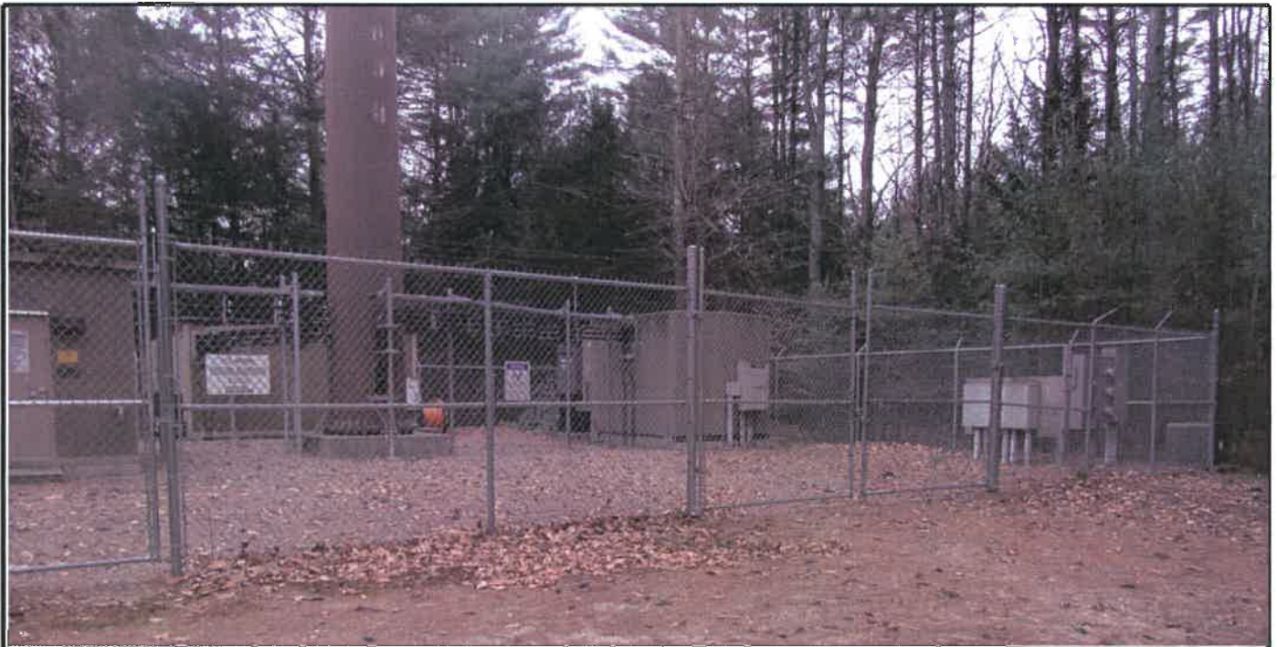
Photo 3 - VIEW EAST TOWARD EXISTING TOWER COMPOUND
