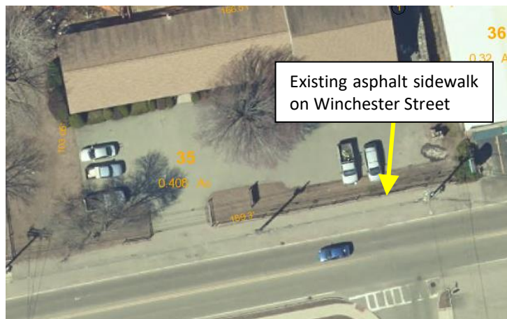
Figure 2. Aerial image showing the location of the existing sidewalk that would be disrupted by the proposed curb cut.
