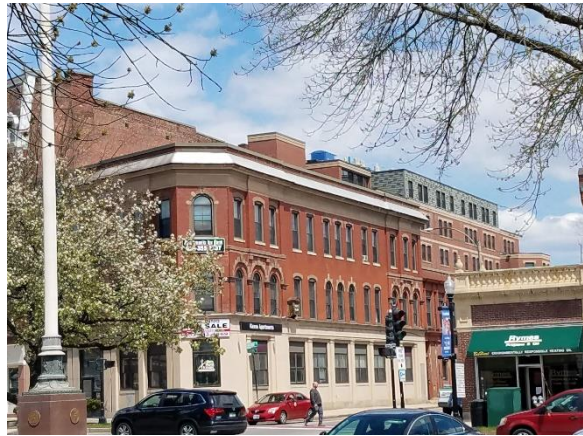
Figure 4. View of the Roxbury Street facade of the Central Square Terrace building from Main Street. Mini splits and blue enclosure for mechanical equipment are visible above the mansard roof.
