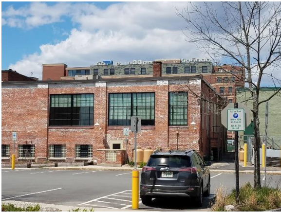
Figure 3. View of the Roxbury Street facade of the Central Square Terrace building from Church Street. Mini split units are visible above and to the right of the mansard roof.
