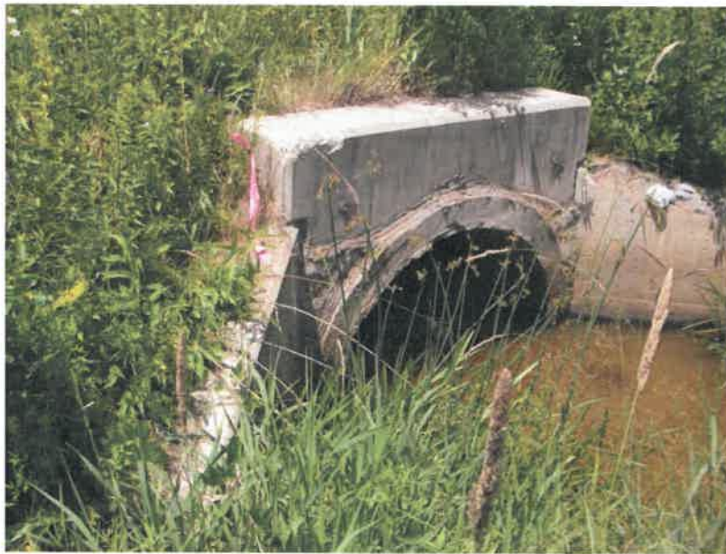
Photo 8 – PEM1Ed Wetland Drainage Inlet (6/30/2016)
