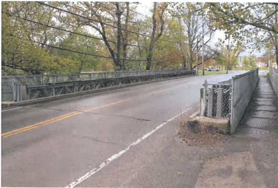
Photo 4 – Island Street Bridge Facing South (5/15/2019)
