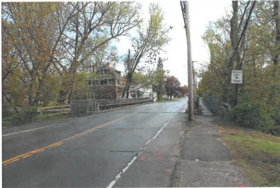
Photo 1 – Island Street Bridge (127/068) Facing North (5/15/2019)
