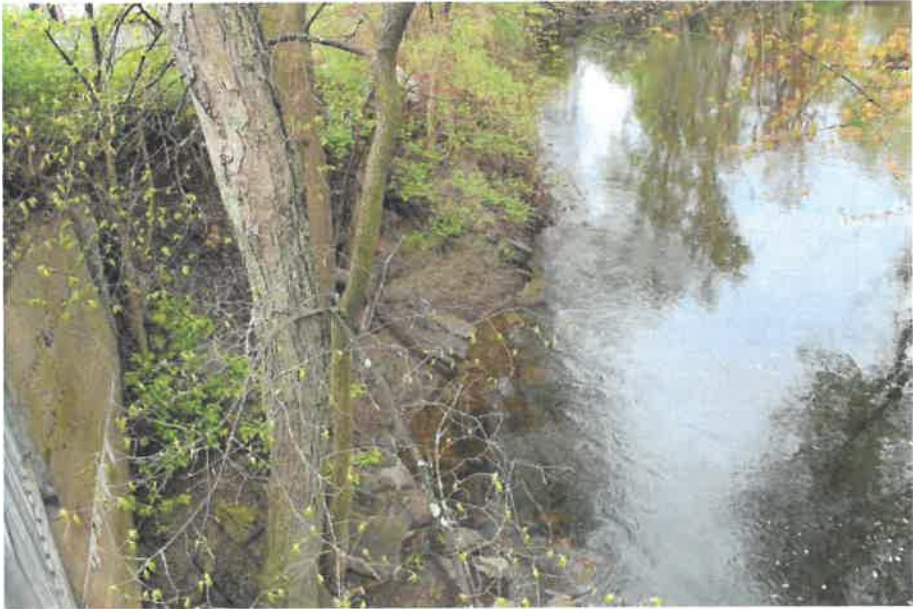
Photo 6 – Retaining Wall in Southwest Bridge Quadrant (5/15/2019)
