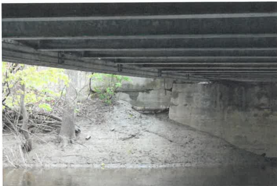
Photo 2- Northern Bridge Abutment and Adjacent Retaining Wall (5/15/2019)
