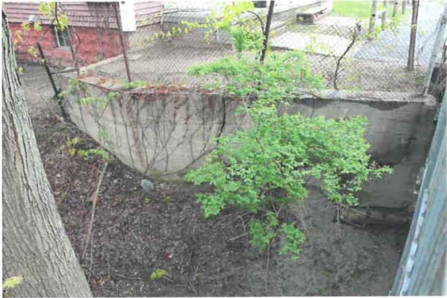
Photo 5 – Retaining Wall in Northwest Bridge Quadrant (5/15/2019)
