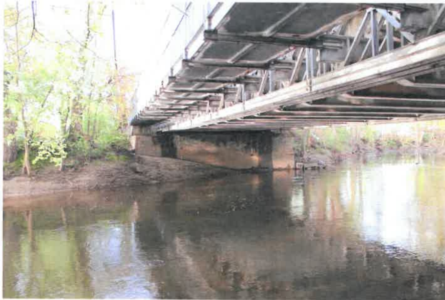
Photo 3 – Ashuelot River and Southern Bridge Abutment Facing Southwest (5/15/2019)
