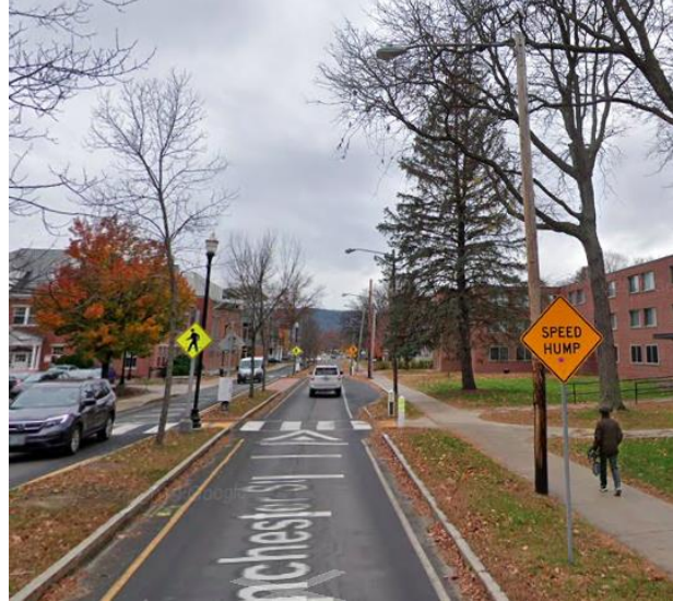
Elevated Crossing at Winchester Street in Keene; Source: Google Maps
