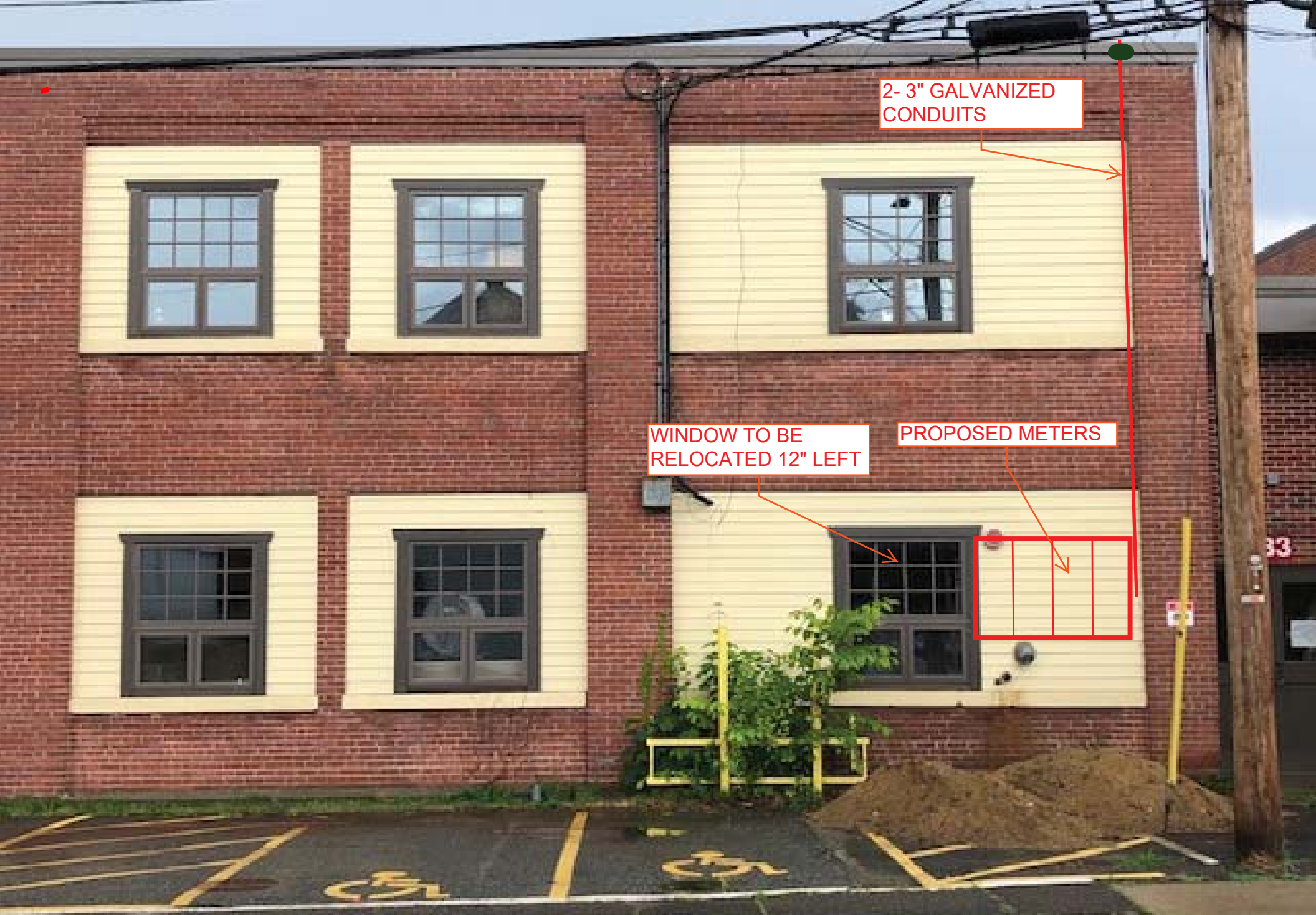
A Rendering Showing the Window to be Relocated & the Proposed Meter & Conduit Locations Along Spring Street
