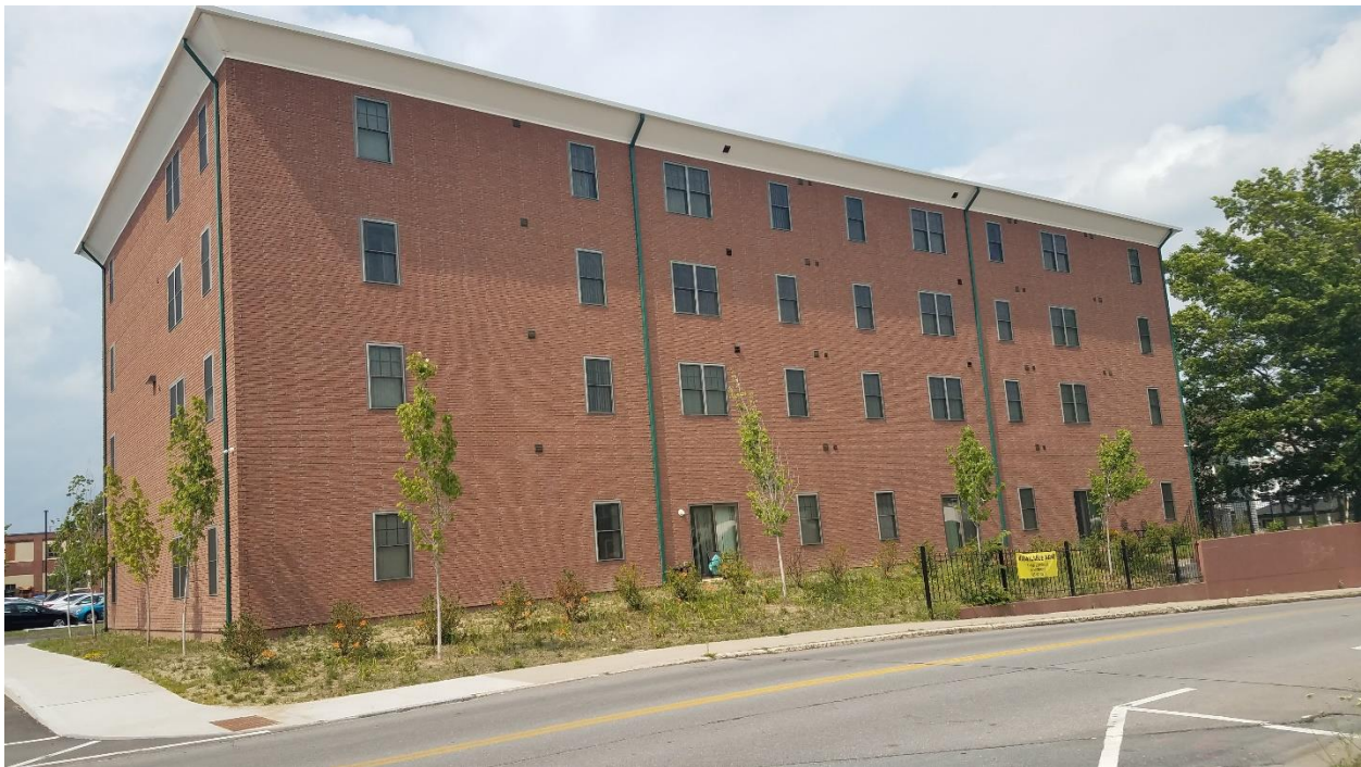
Figure 4. Photo of the south building facade facing Roxbury Street, taken on July 8, 2020.
