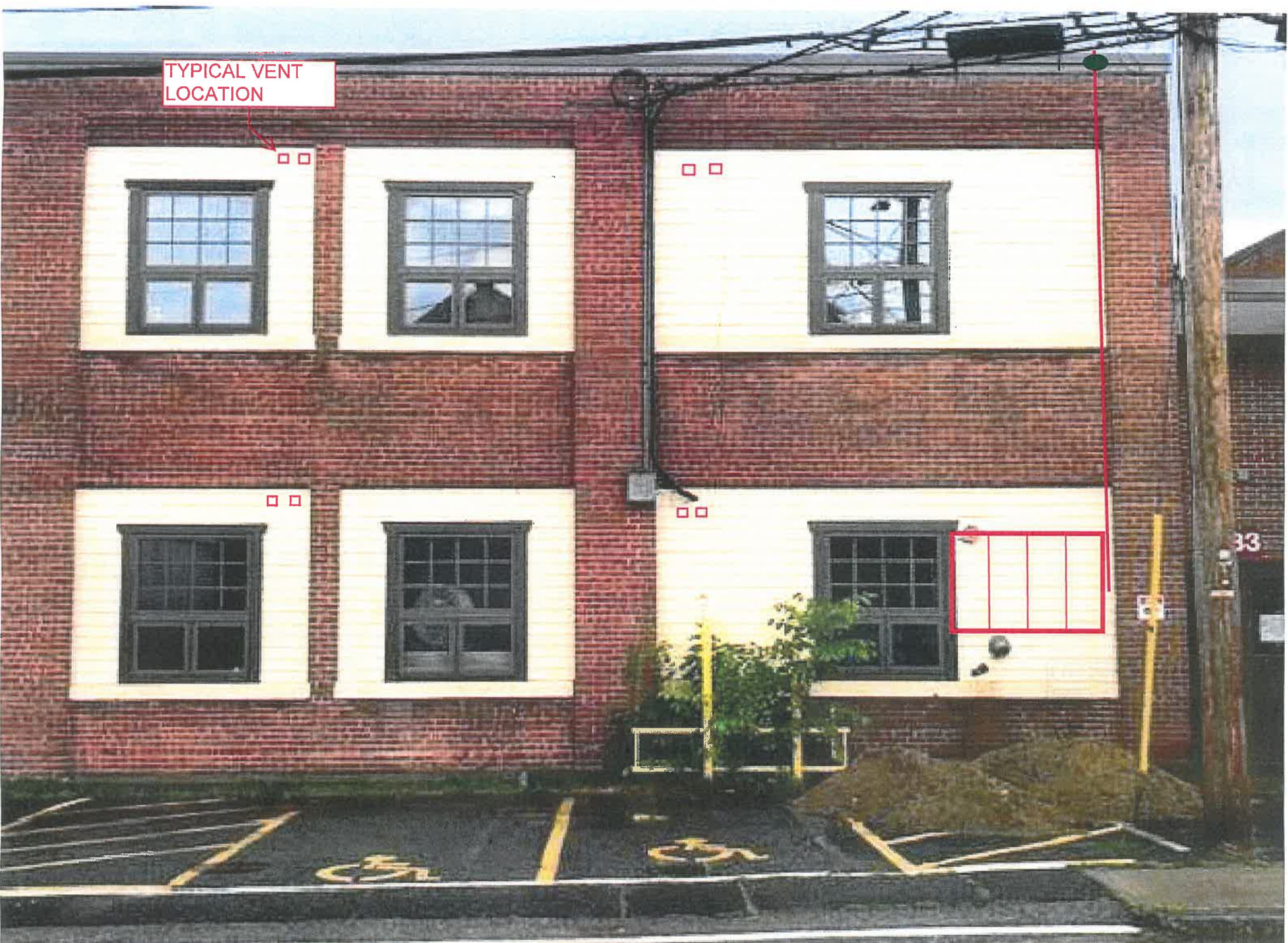
A Rendering Showing the Proposed Vent Penetrations Along Spring Street
