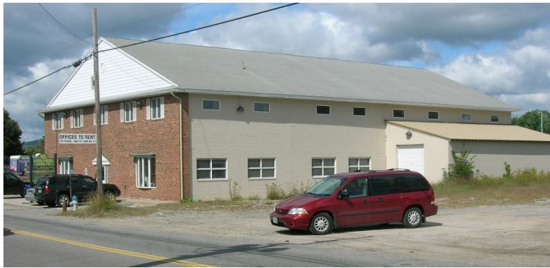
Figure 3. The eastern façade of the building located at 85 Emerald Street, where the Rapid Shutdown Switch will be installed. Photo taken 9/10/09.
