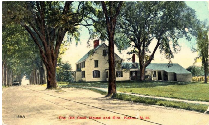
Figure 2. Historic photo showing the Noah Cooke House and the old “Cooke Elm” located at 136 West Street (now the location of People’s United Bank at 122 West Street). Image source: Historical Society of Cheshire County.
