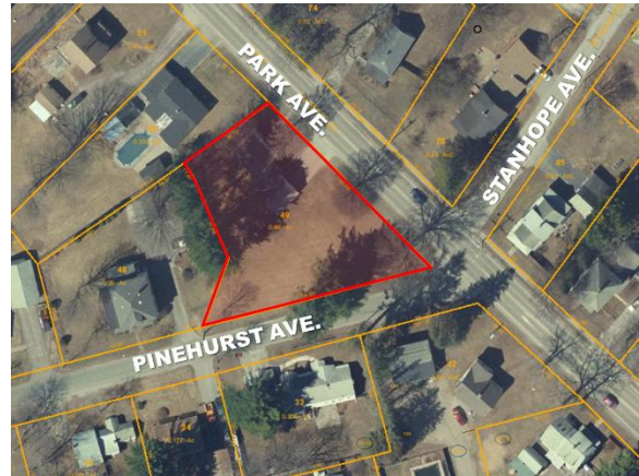
Figure 1. Aerial view of the property located at 366 Park Ave. (outlined in red).
