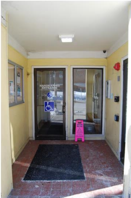
Sidewalk ADA Entrance Existing
