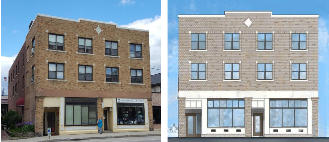
Figure 4. Photo submitted by the Applicant showing the existing Bennett Block Storefront (left) and a rendering showing the proposed storefront (right).
