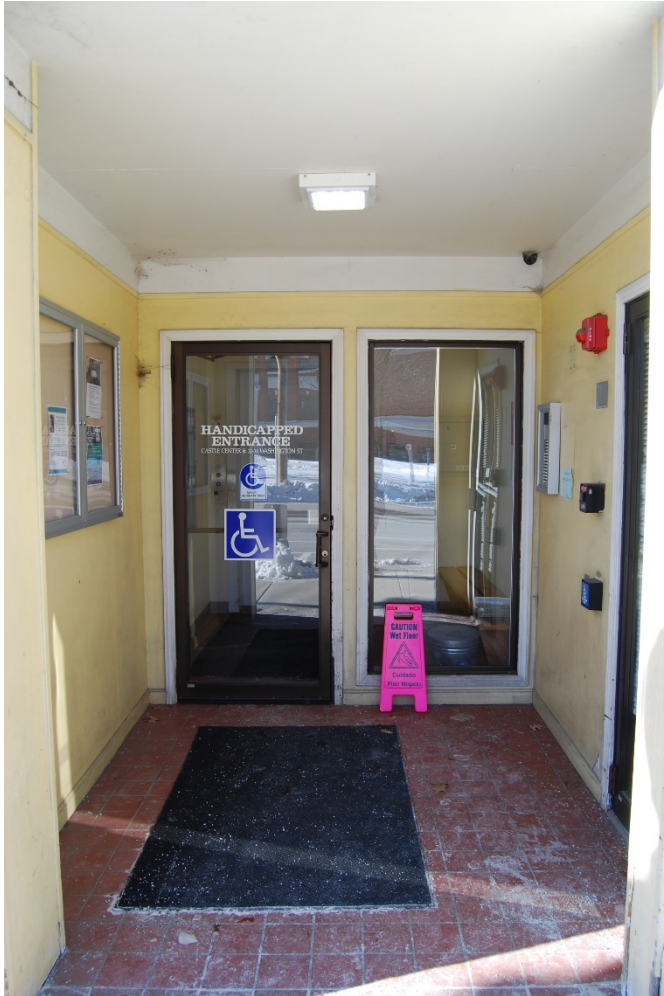
Sidewalk ADA Entrance Existing
