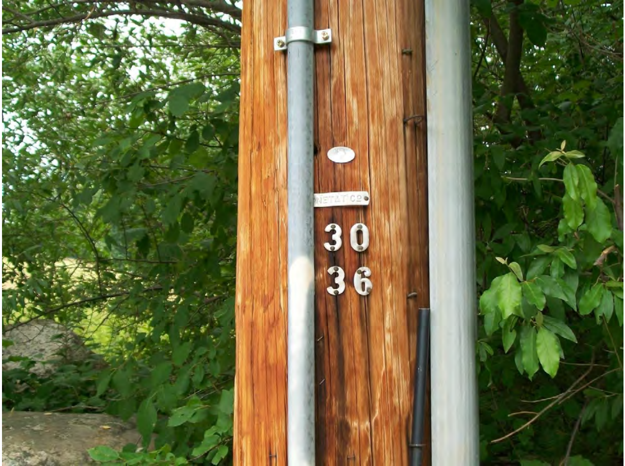
Riser pole on the west side of the underpass
