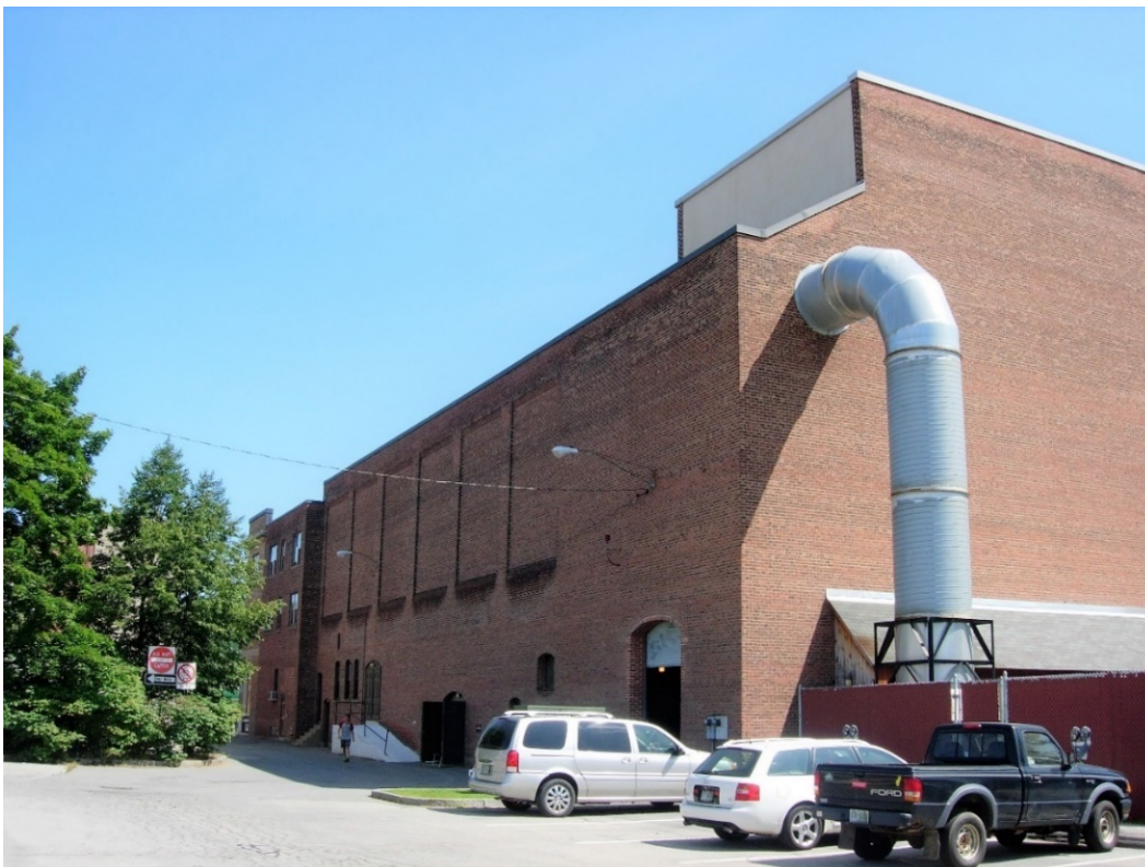
Figure 2 – Existing Stage House view from public parking
