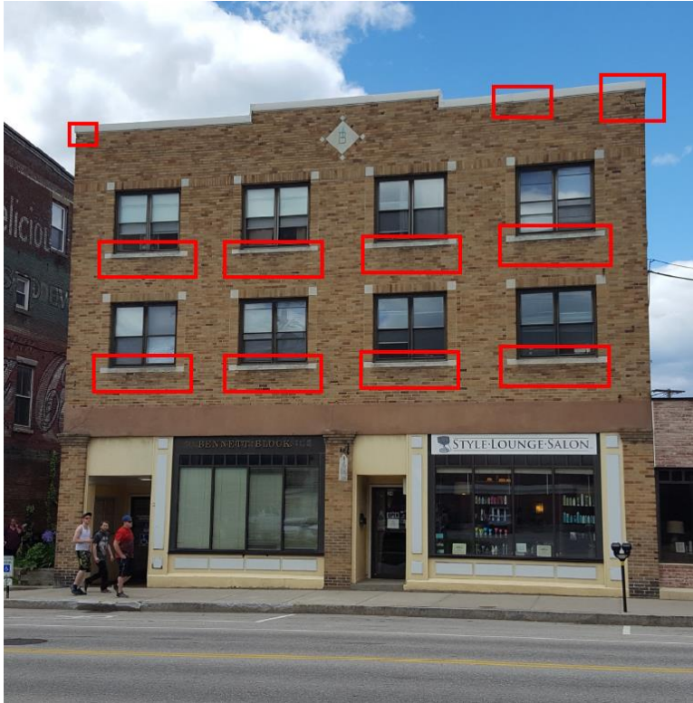
Figure 2. (Left) Photo submitted by the Applicant showing the proposed areas of masonry repair on the primary façade of the building.
