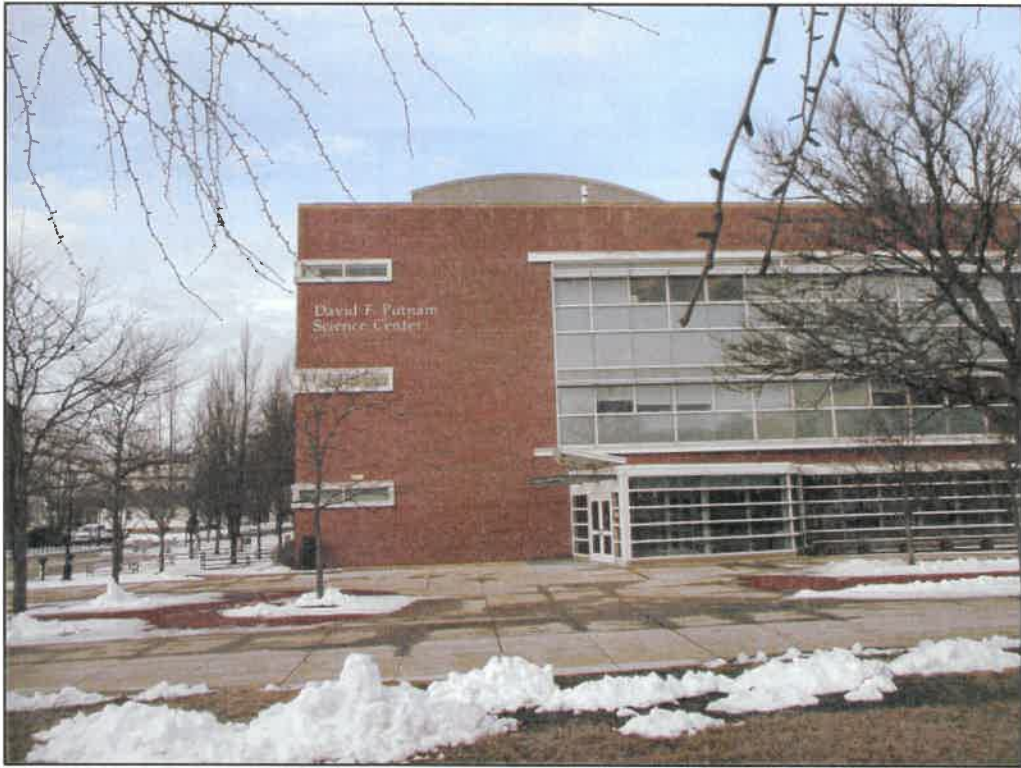
Photograph 1 – Subject property, facing north.
