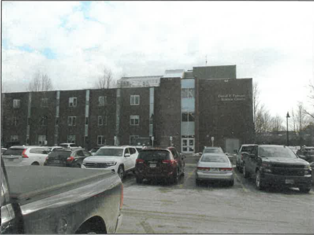
Photograph 3 – Subject property, facing south.
