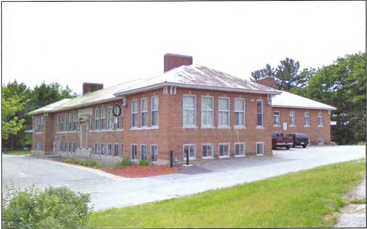
Photo 1: View looking SW-W at main façade and northeast elevation of original school
