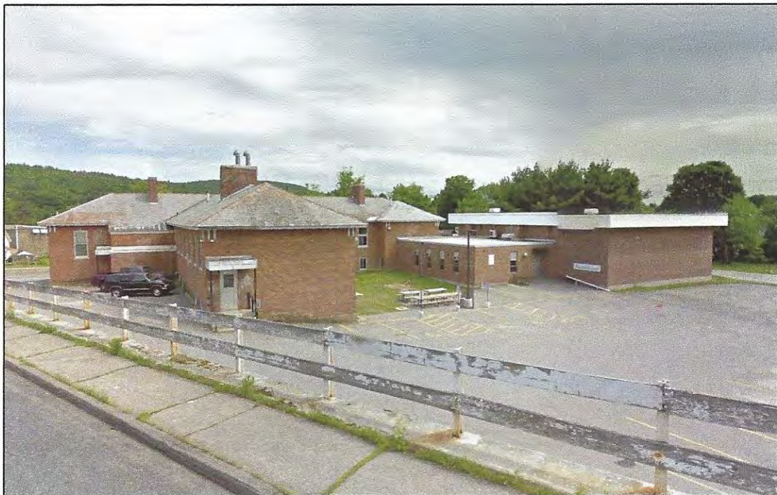
Photo 3: View looking SE from Woodbury Street. Rear elevation of original building at left and c.1970 addition at right.
