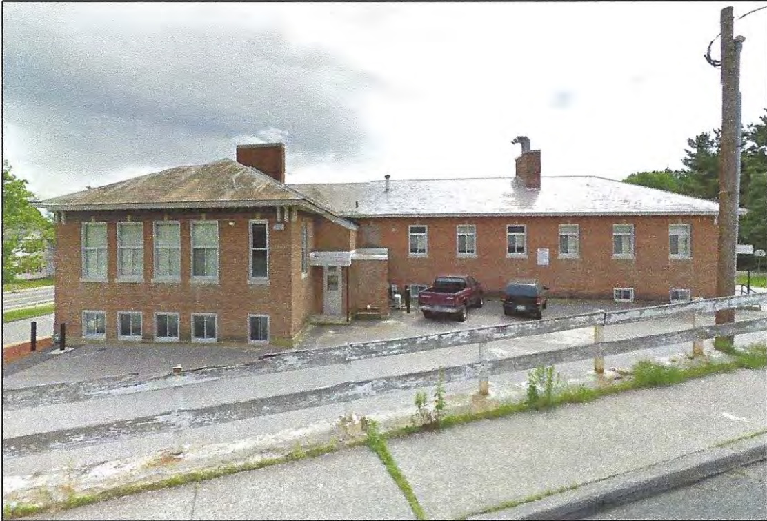
Photo 2: View looking SW from Woodbury Street at original school building.
