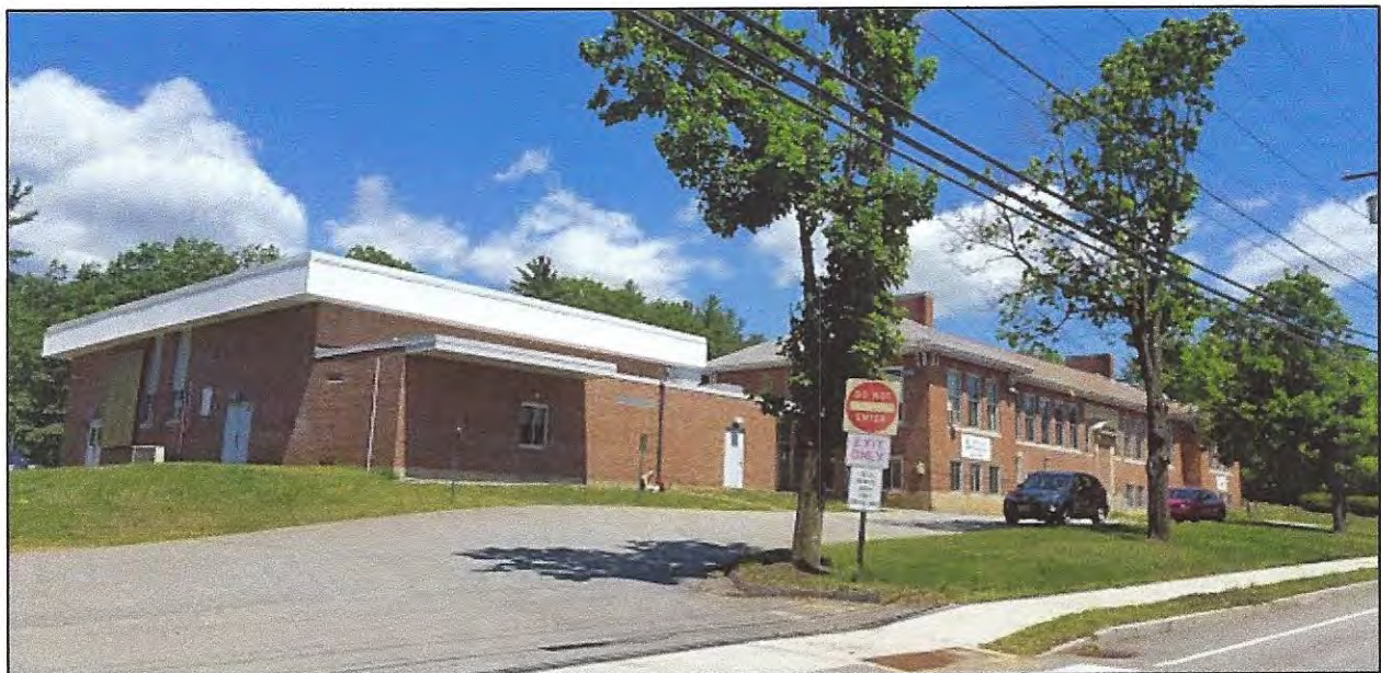
View of original building with c.1970 addition at left.
