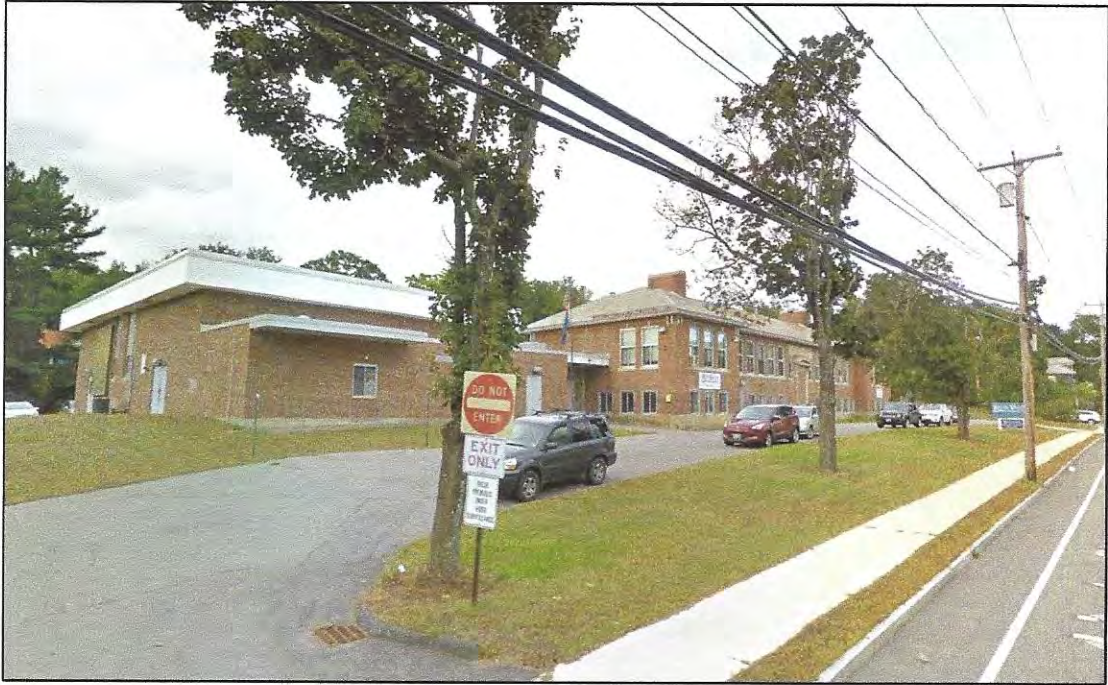
Photo 4: View looking north from Washington Street. C.1970 addition at left and original school building to right.
