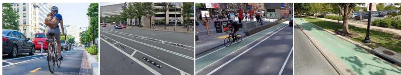
Fig. 3. Examples of protected bike lanes with light separation, from left to right: 15th Street NW, Washington DC, separated with posts and parked cars; Pennsylvania Ave NW, Washington DC, separated with parking stops; 7th Avenue, New York, separated with continuous low curb and grade, immediately adjacent to the road; 1st Street NE, Washington DC, separated with continuous low curb.
