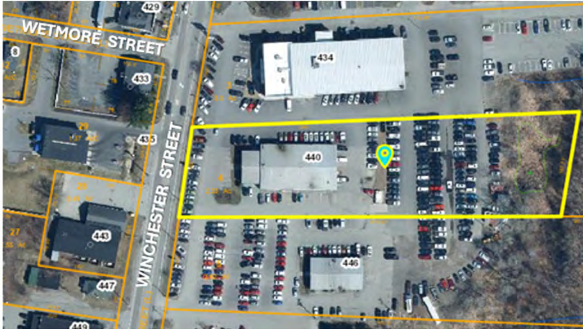
Figure 1. Aerial imagery from 2020 showing the parcel at 440 Winchester St.
