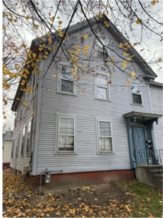
Figure 4. A photo of the existing building exterior submitted by the applicant.
