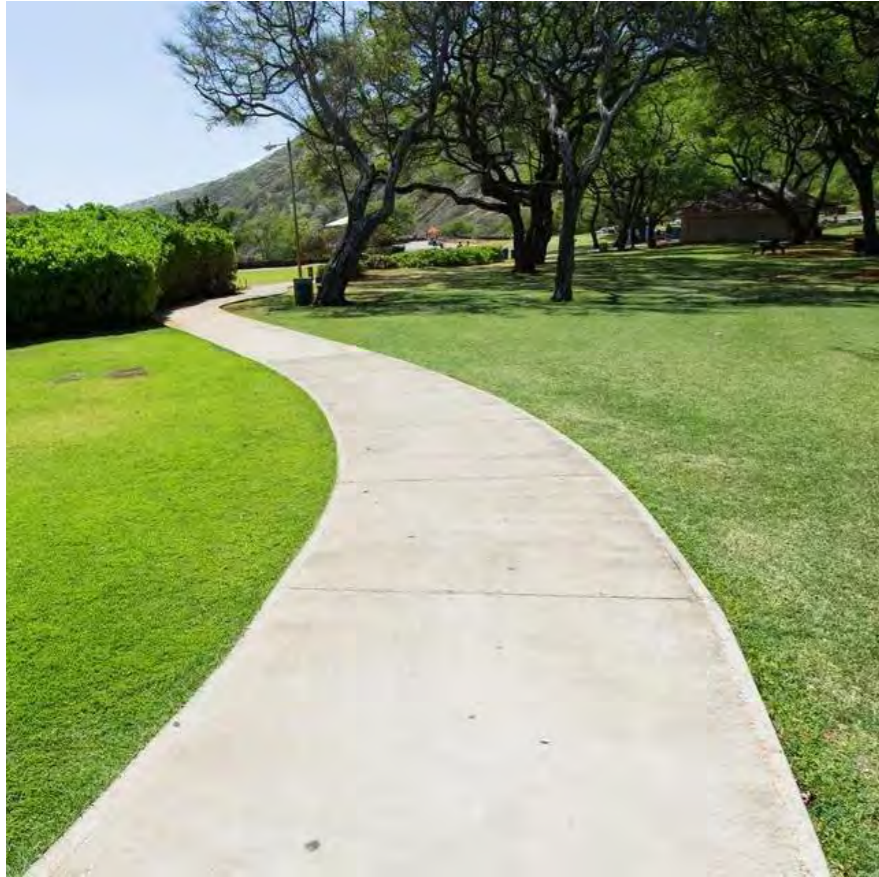
STANDARD CONCRETE (BROOM FINISH AND/OR EXPOSED AGGREGATE)
