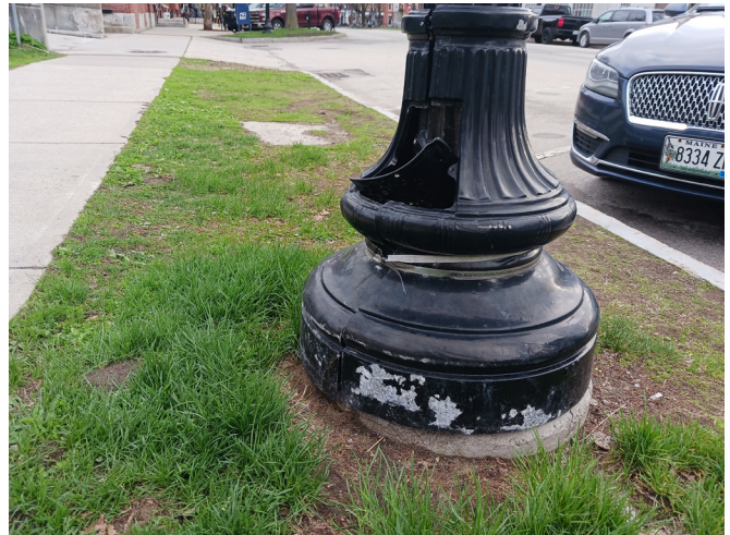
Light Pole Base
