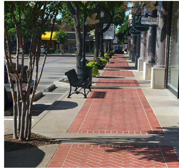
Stamped concrete - colors and pattern can vary
