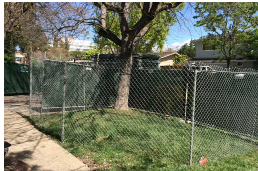
Chain-link fence tree protection
