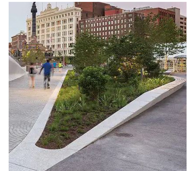
Precast concrete - flush curb to seat wall transition
