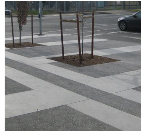
Sandblasted for subtle texture and pattern change
