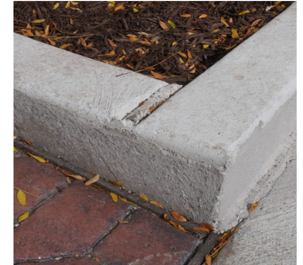
Cast-in-place concrete curb
