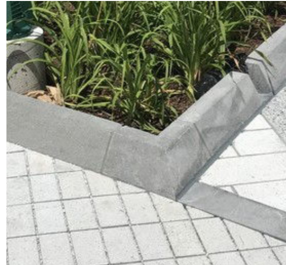
Tapered granite curb
