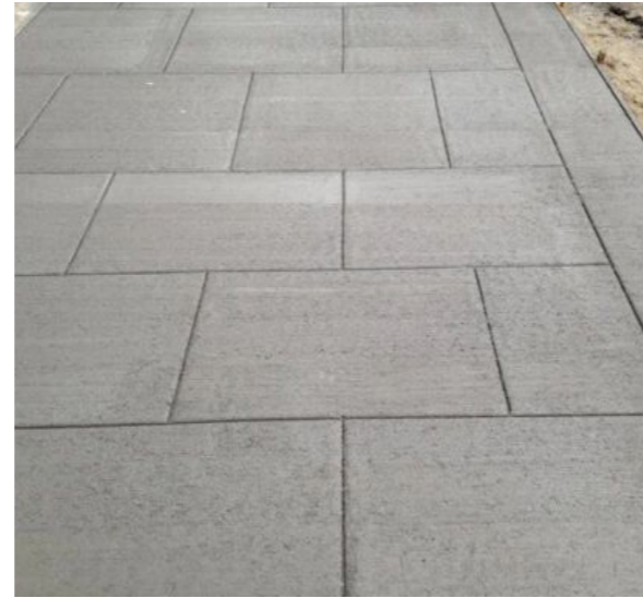
Standard broom finish, scoring pattern
