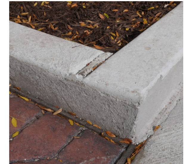
Cast-in-place concrete curb
