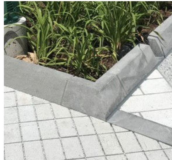
Tapered granite curb
