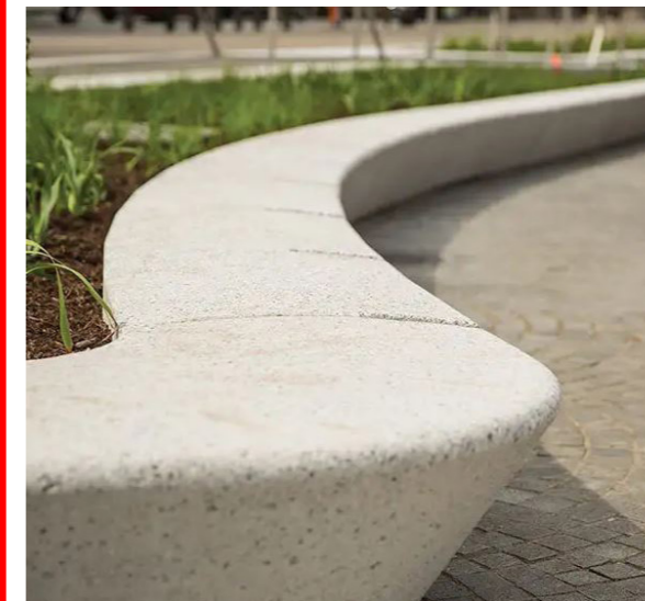
Precast concrete seatwall
