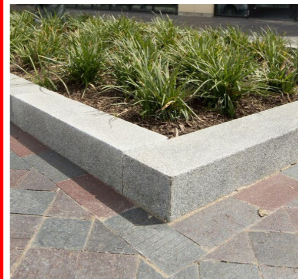
Vertical granite curb
