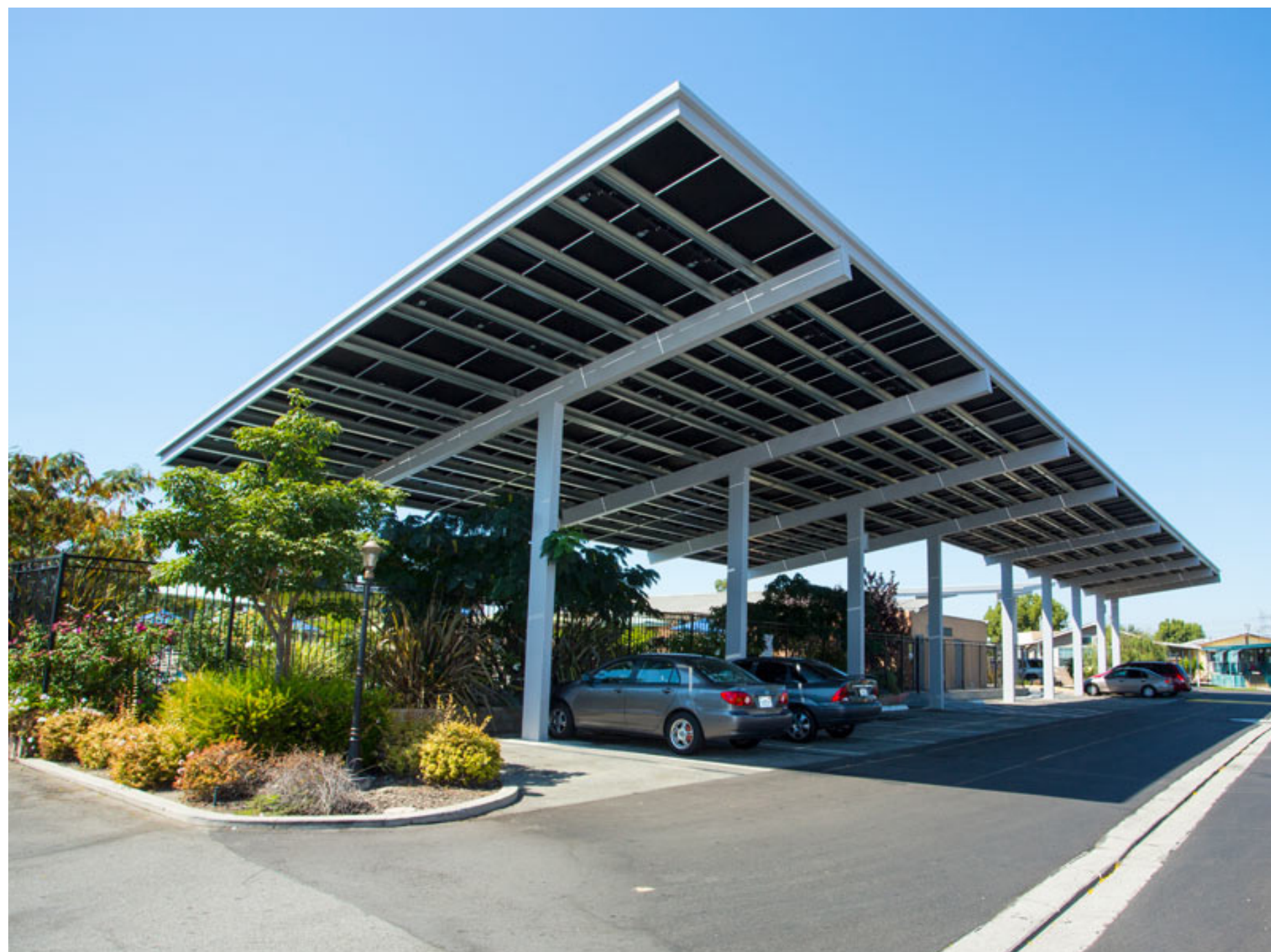
Solar Structure over Parking
