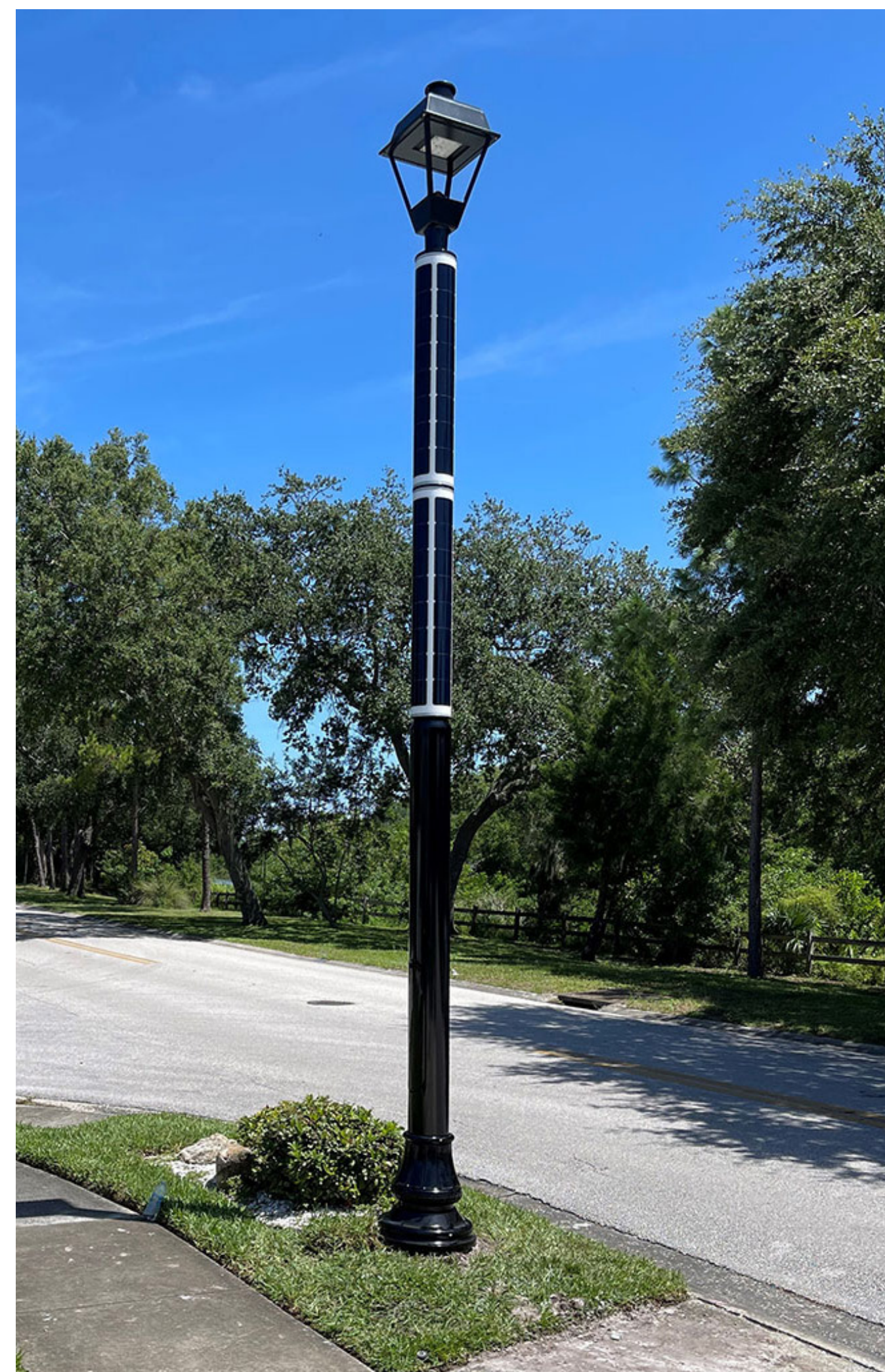
Solar Street Light
