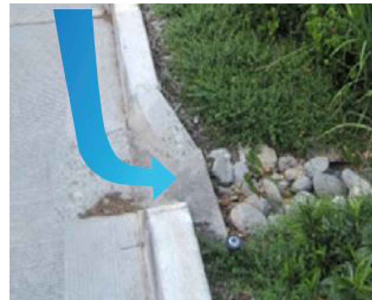
An angled curb cut with a graded
