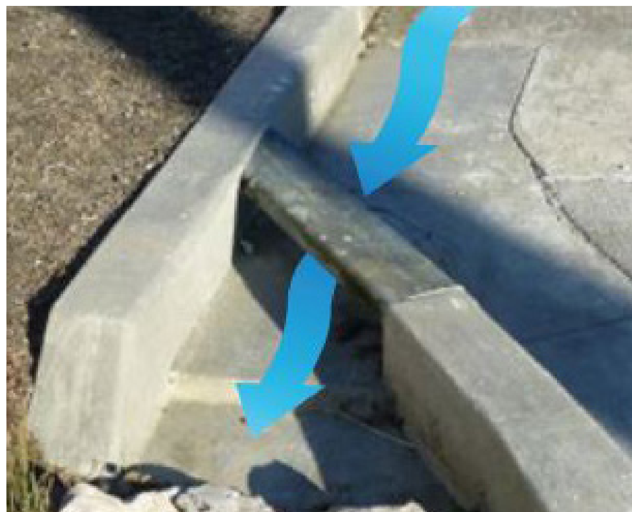
Metal extension inlet structure provides a wide opening for stormwater flow
