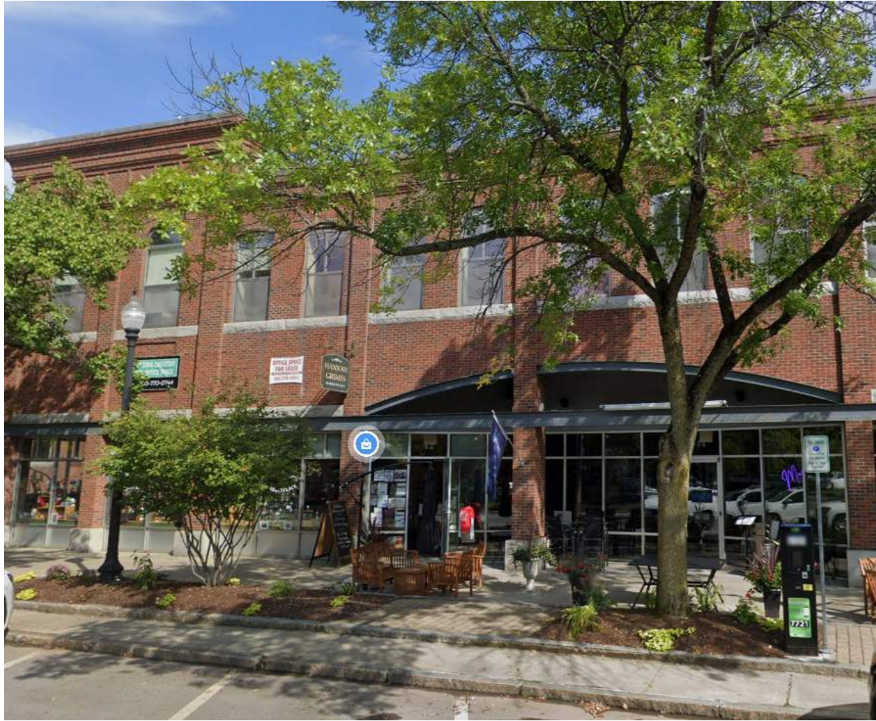
Existing - Planting Bed with Trees
