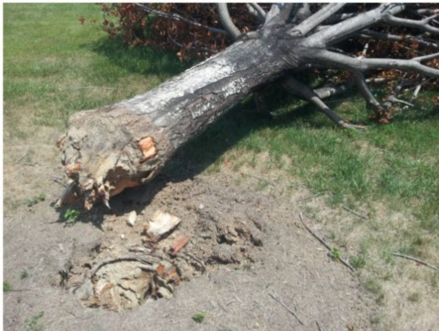
Example of tree failure from girdling roots.
