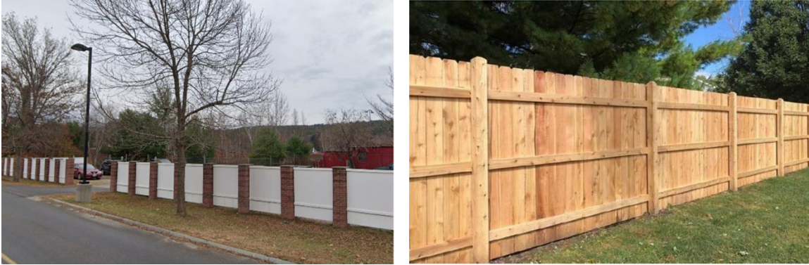
Figure 5. Images of existing vinyl fencing with brick columns on the 122 Water St. site (left) and proposed solid cedar fencing for the perimeter of the 124 Water St. site (right).
