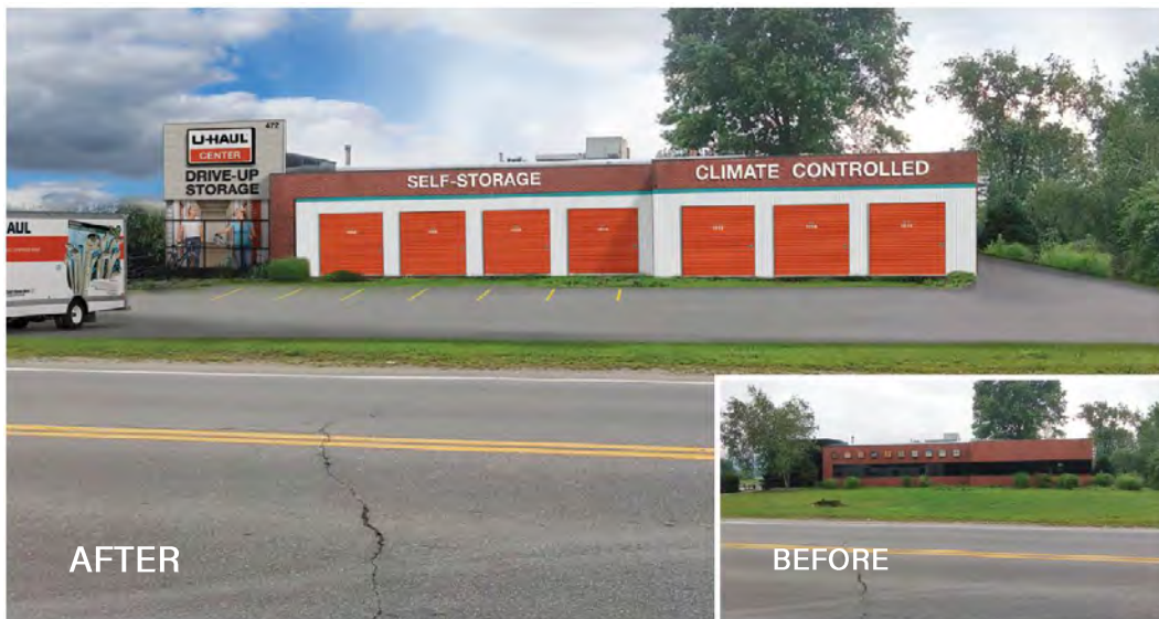
Figure 4. Image of the proposed rendering for the Winchester Street facade. The Applicant proposes to replace the windows and brick exterior with metal siding with bright orange, faux self-storage doors that match the corporate U-Haul aesthetic.
