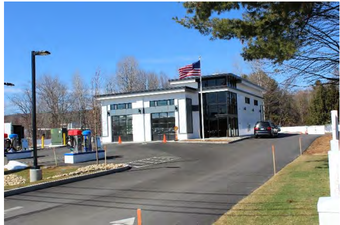
Figure 1. Image of the Mint Carwash building located at 435 Winchester Street.
