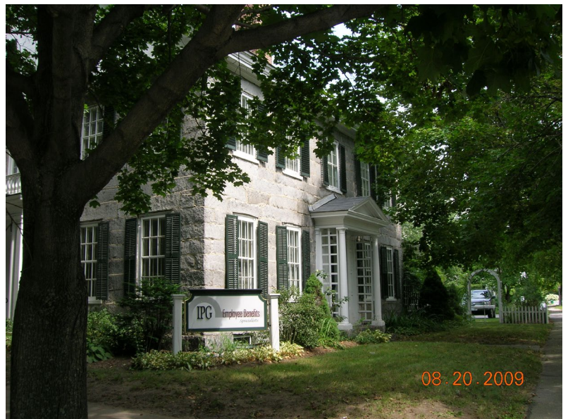
Figure 2: Facade at 85 Washington Street
