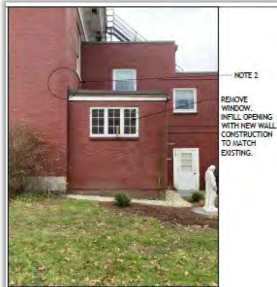
Figure 2. Kitchen window proposed to be removed
