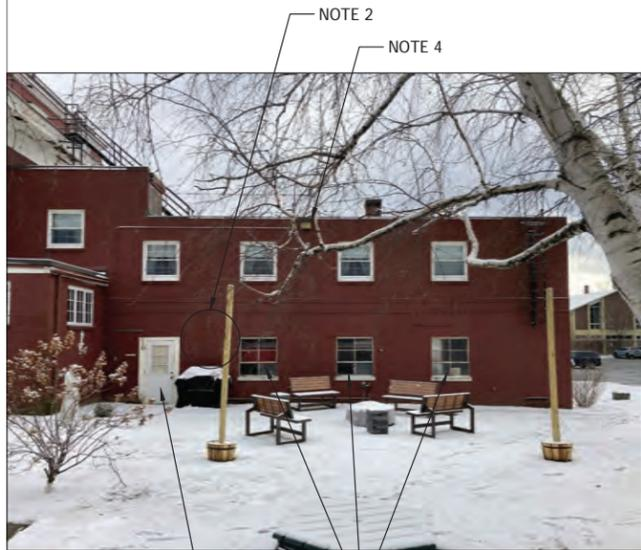
NEW INSULATED ENTRY DOOR (THERMA-TRUE; FIBERGLASS OR STEEL) AND WOOD FRAME, PAINTED
