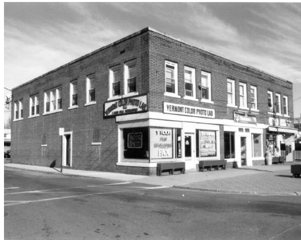
Figure 2. Photo of the south and east facades of the 147 Main Street building, taken in the fall of 2002.
