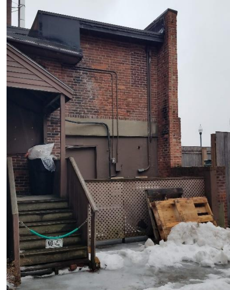
Figure 4. Photo of the existing fenced-in area where a generator is proposed to be installed on the 35-43 Main Street property. Date of photo: 2/1/22.
