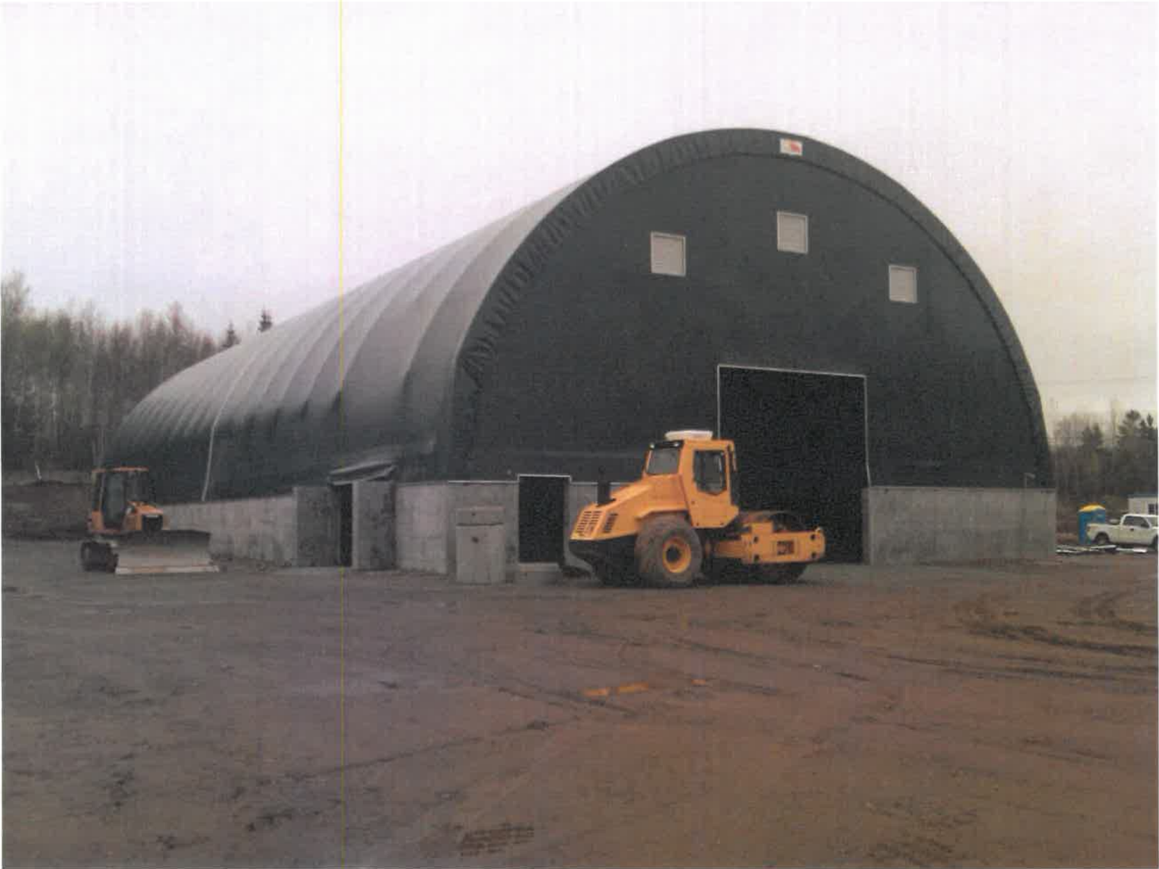
SALT SHED TYPICAL, GREEN CANOPY
