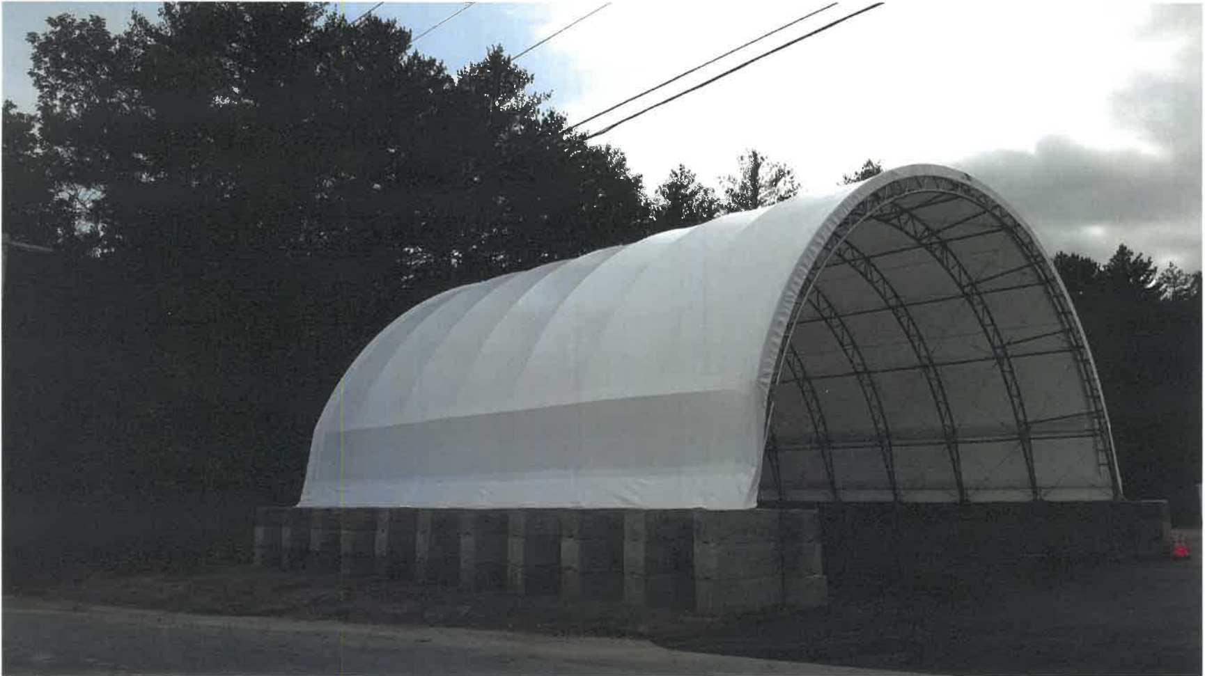
SALT SHED STRUCTURE, CONCRETE BLOCK FOUNDATION
