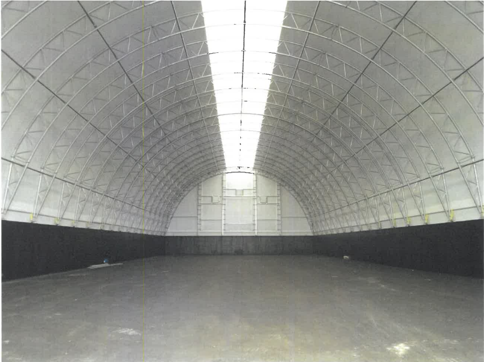
SALT SHED STRUCTURE, WHITE STRIP FOR NATURAL LIGHTING
