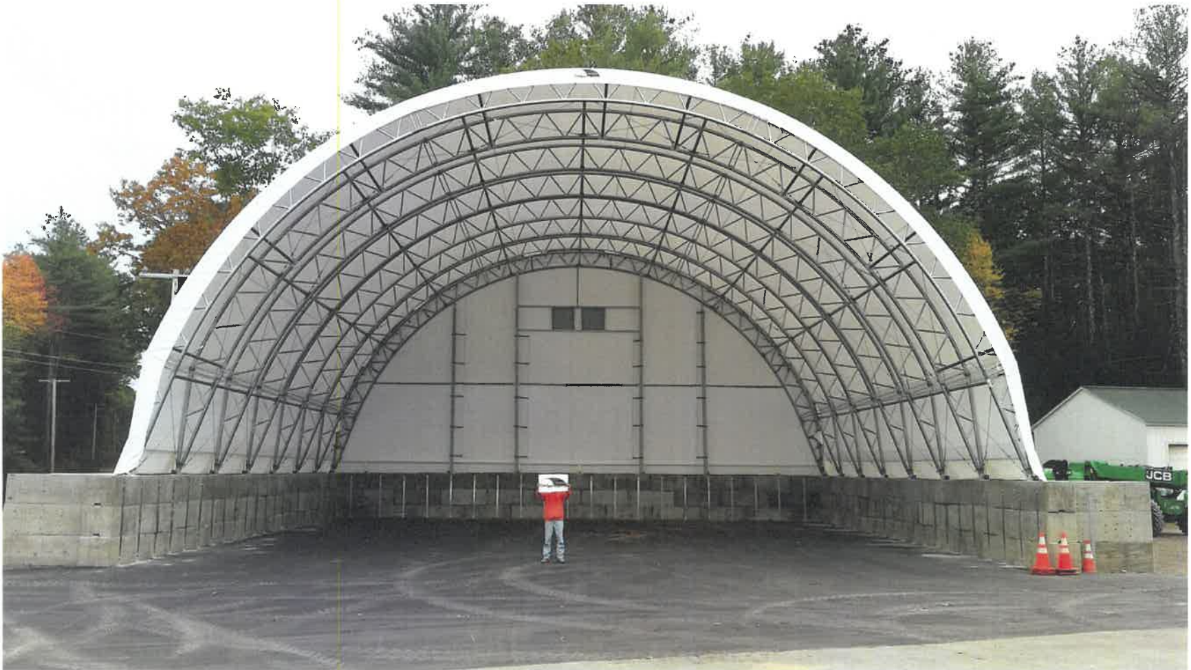
SALT SHED STRUCTURE, BACK WALL DETAIL
