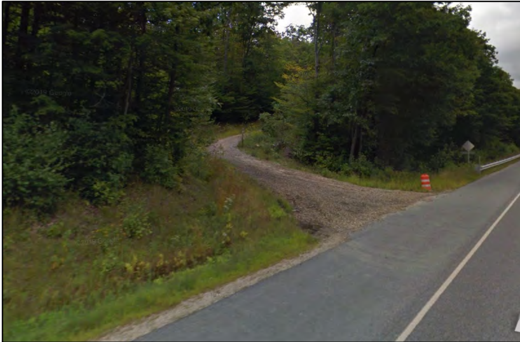
Photo 5. Existing entrance drive.
