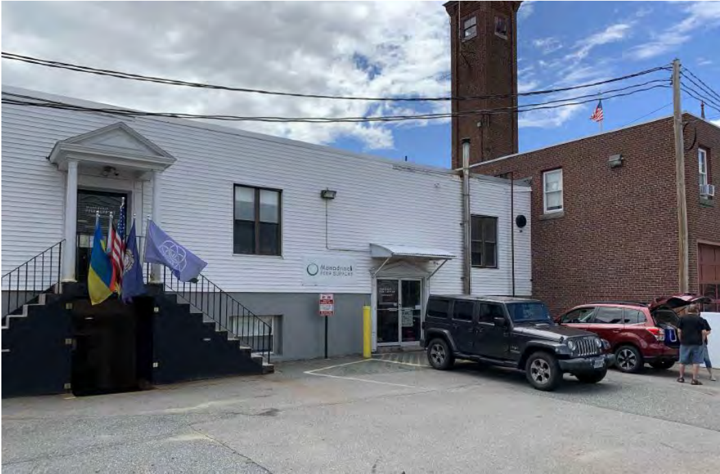
Figure 3. Photo submitted by the applicant that shows the existing MPS building and the proposed designated smoking area.
