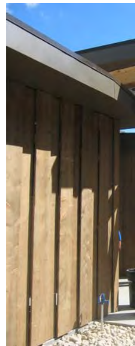
Figure 2. Skip/lap fencing.
