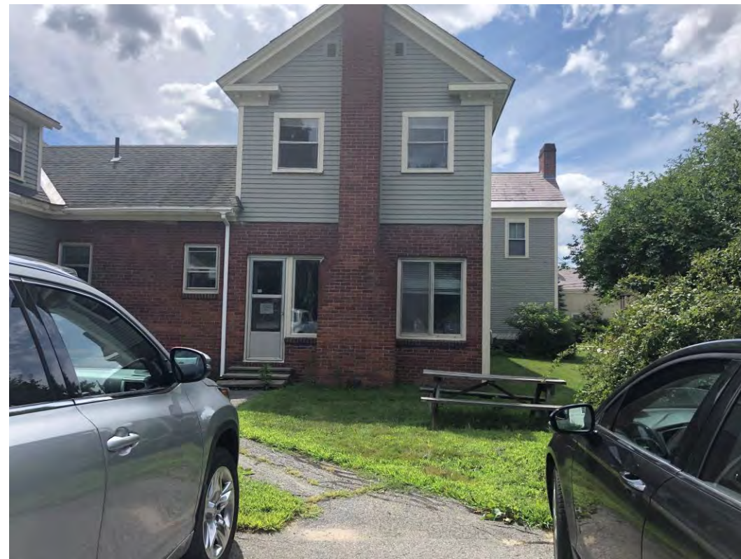
Photo Above: View of the back of the building at 39 Summer Street. Photo taken facing south.
