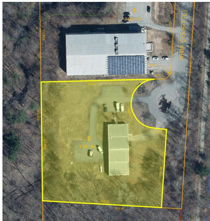
Fig 1: Aerial view of 7 Krif Court
